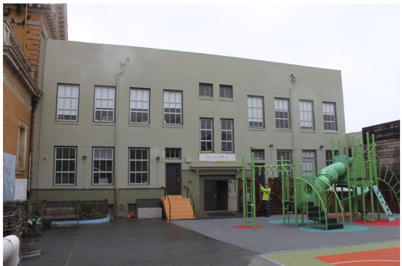
FIGURE 45. SCHOOL: REAR (SOUTH) ELEVATION AND SCHOOL YARD, 2016.
