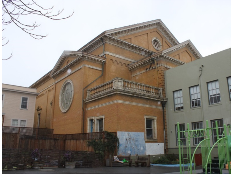
FIGURE 12. CHURCH: REAR, EAST ELEVATION FROM INTERIOR OF LOT, 2016.
