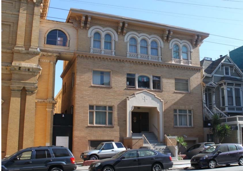
FIGURE 38. RECTORY: MAIN (WEST) ELEVATION FROM FILLMORE STREET, 2015.
