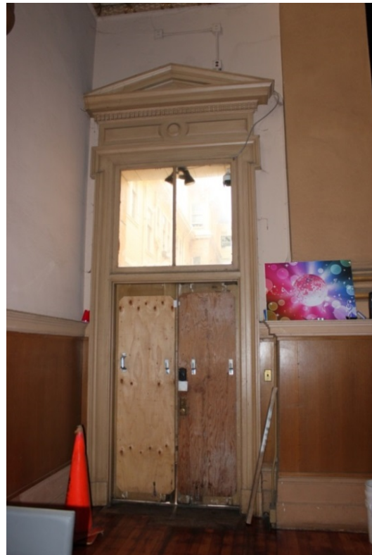
FIGURE 31: CHURCH: NAVE, SOUTH TRANSEPT ENTRY TO ALLEY, 2016.
