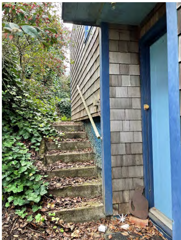
651 Duncan Street, entry and east elevation, view southwest, 2020 Source: YA Studio
