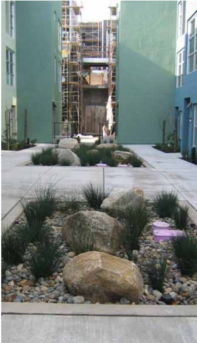
Linked bioretention cells are a central part of the design for the Glashaus development in Emeryville, CA.
