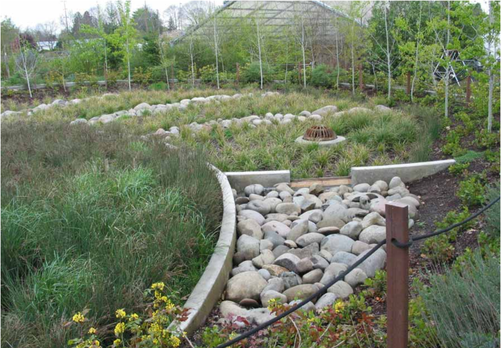
A rain garden at Glencoe Elementary in Portland, Oregon reduces stormwater flows to Portland's collection system.
