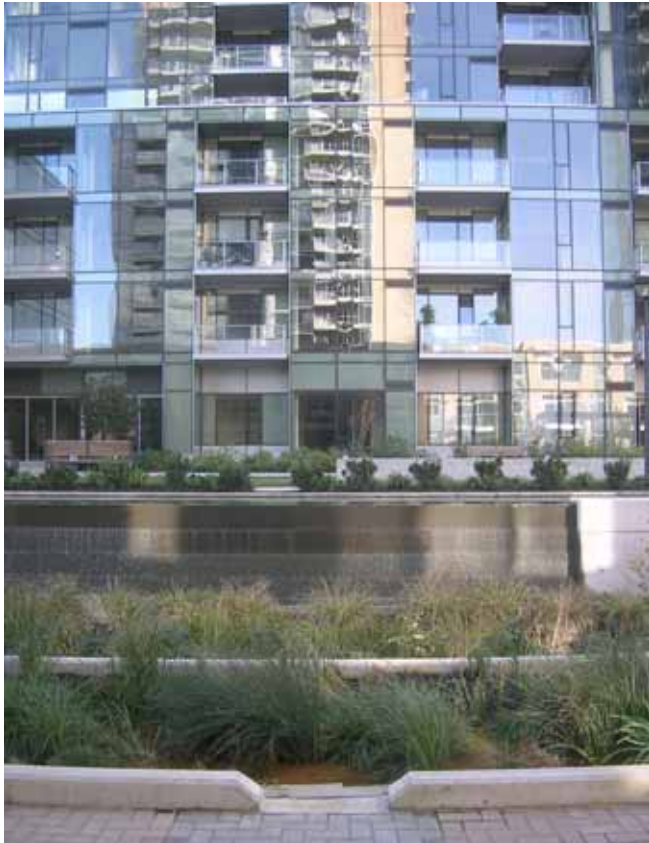
Stormwater treatment facilities enhance public spaces in Portland's South Waterfront redevelopment area.
