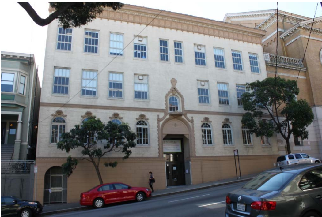
FIGURE 43. SCHOOL: MAIN (NORTH) ELEVATION, LOOKING SOUTH FROM FELL STREET, 2015.
