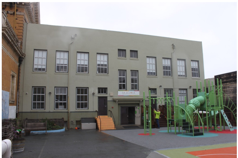
FIGURE 45. SCHOOL: REAR (SOUTH) ELEVATION AND SCHOOL YARD, 2016.
