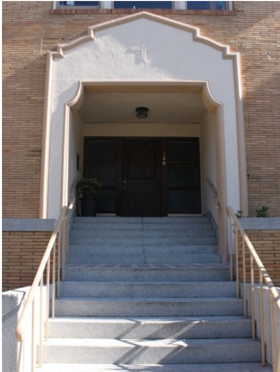
FIGURE 39 (LEFT). RECTORY: MAIN ENTRANCE, 2015.
