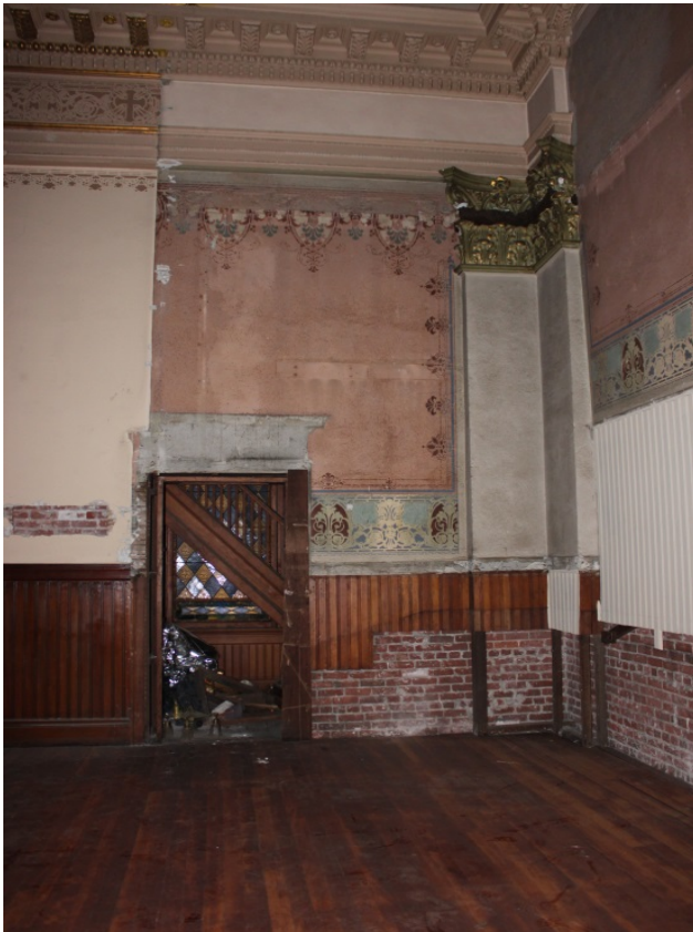
FIGURE 22. CHURCH: CHOIR LOFT, SOUTHWEST CORNER AND DOOR TO CONNECTOR TO RECTORY, 2016.
