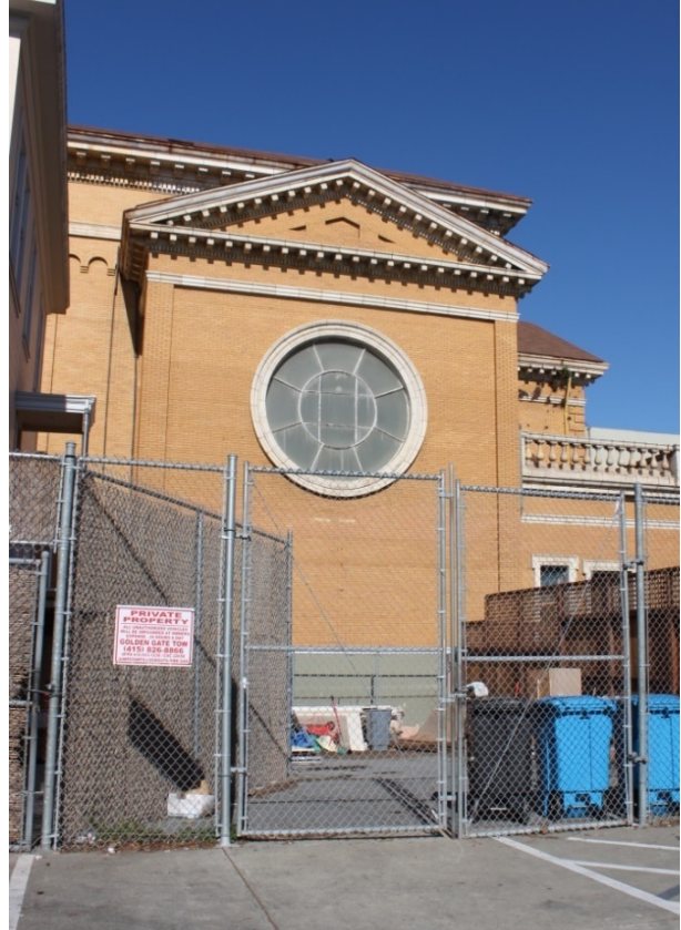
FIGURE 11. CHURCH: SOUTH TRANSEPT AND SACRISTY LOOKING NORTH FROM PARKING AREA OFF OAK ST., 2015.
