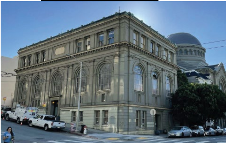
PHOTO OF EXISTING BUILDING:
