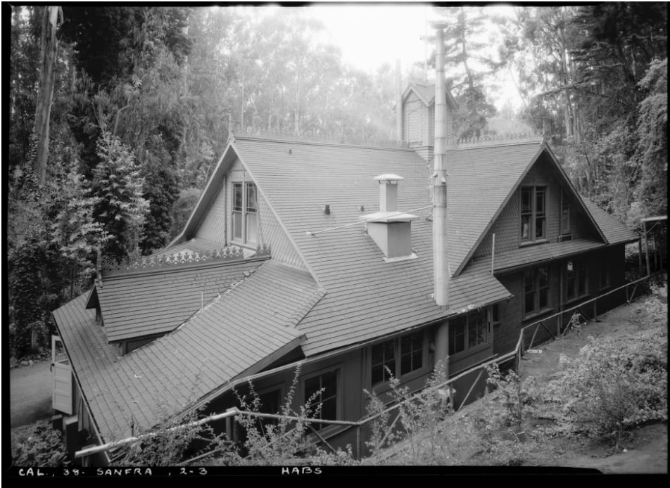
Trocadero Inn, north façade and roof, 1936. Source: Historic American Building Survey, CA-119. Photographer, Robert W. Kerrigan. Accessed via https://www.loc.gov/resource/hhh.ca0738.photos?st=gallery .
