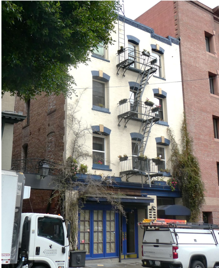
Figure 12. Oblique view 530 Jackson Street. Looking northeast.
