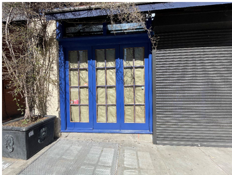
Image 8: Primary façade storefront. (Photo taken by P&T 03/14/2025)
