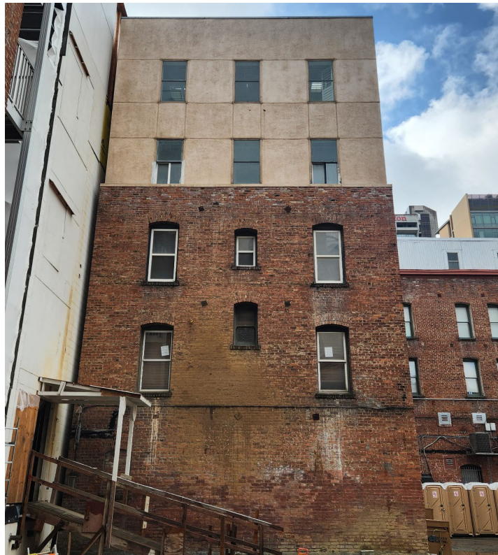
Figure 19: North façade of 530 Jackson Street. Looking south.
