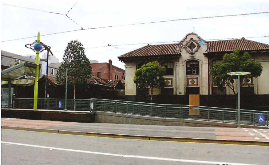
2300 3 rd Street looking westward across 3 rd Street with the 20 th Street light rail stop in the foreground
