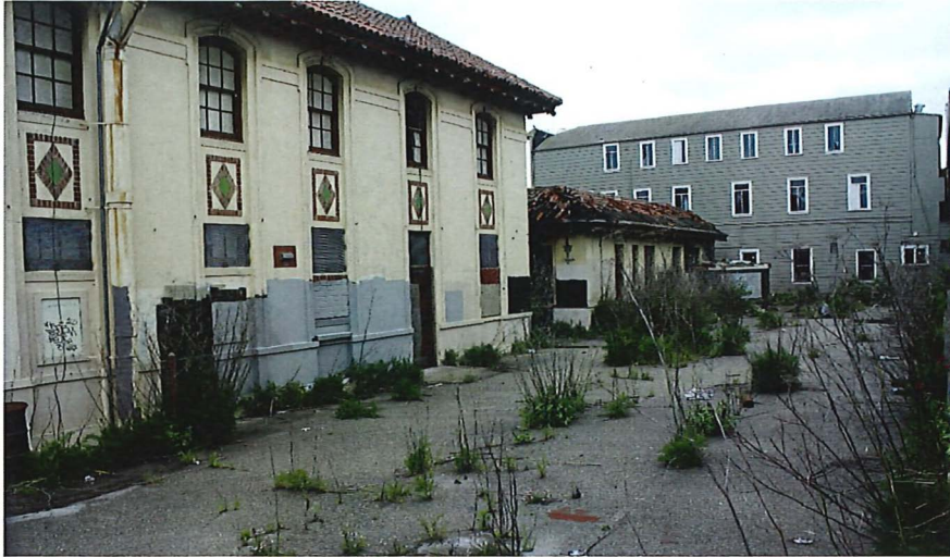
Looking at the rear of 2300 3 rd Street and the paved portion of the site
