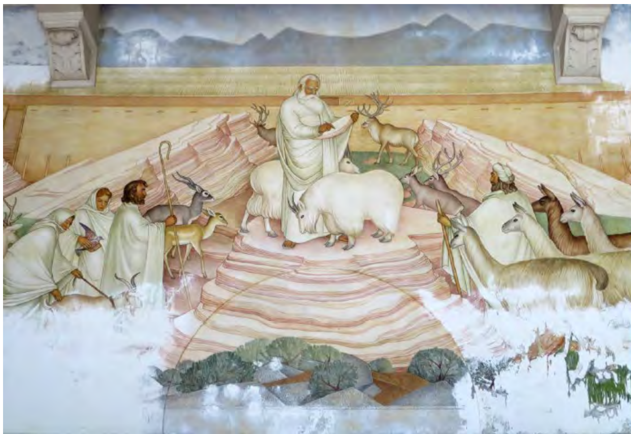
Mother's Building, west wall of main lounge, detail of Loading of the Animals , 2016. Source: Architectural Resources Group, Inc., Mother's Building Conditions Assessment
