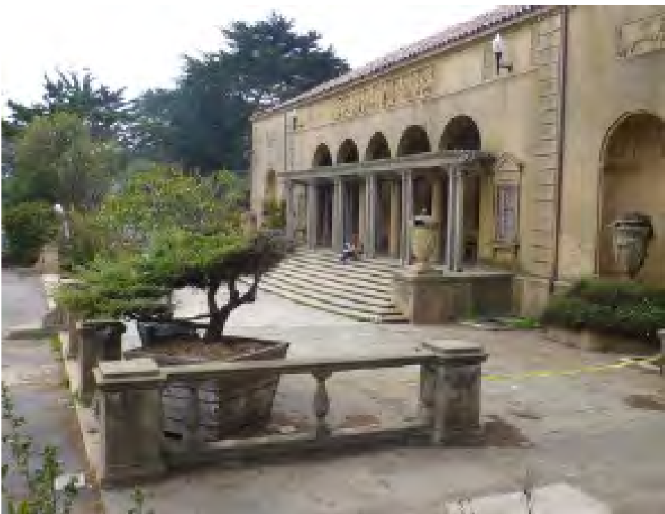
Mother's Building, east elevation and terrace/plaza, view south, 2015. Source: SOHA Engineers
