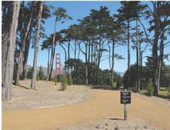
STABILIZED AGGREGATE PAVING
