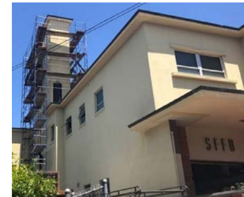
Fire Station - Seismic Hose Tower
