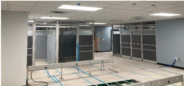
ZSFG 6H Surge – New workstations installation
