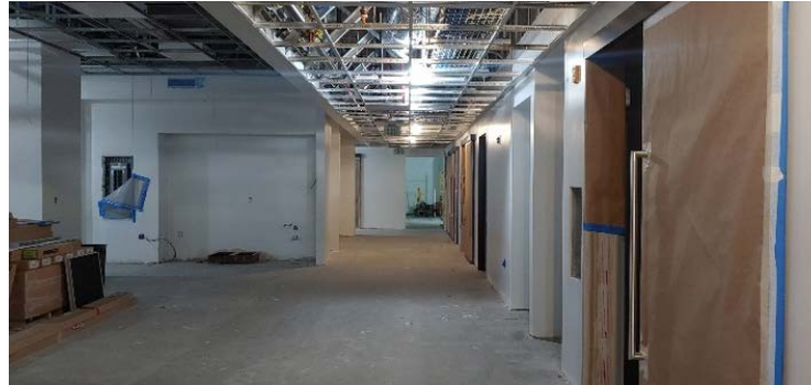
ZSFG Rehab – New Exam Rooms
