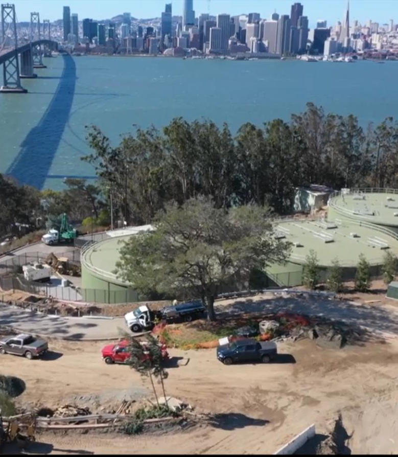
new water tanks
