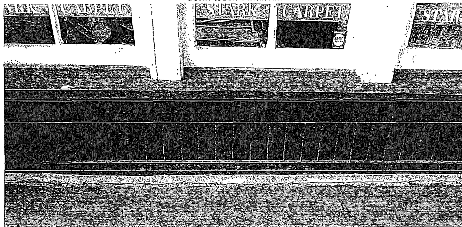
Vertical board bulkhead
