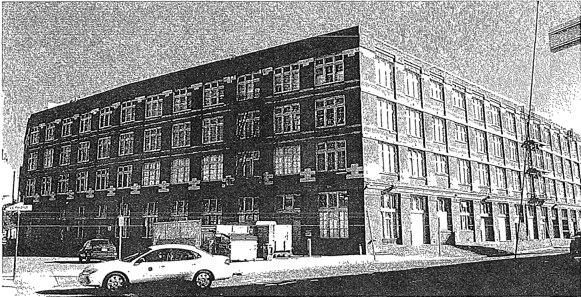
Northwest (l) and west (r) facade
