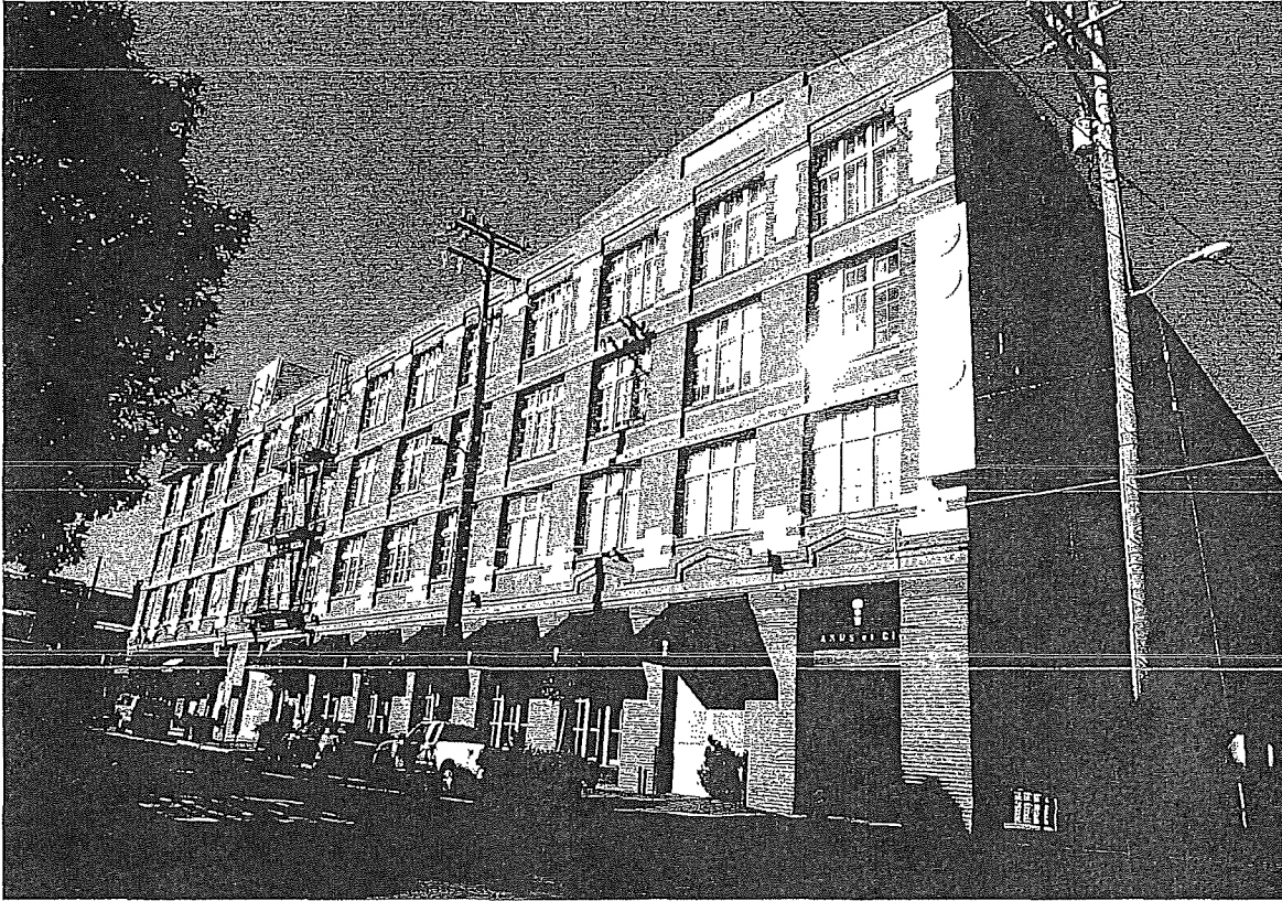
South facade (l), east facade (r)
