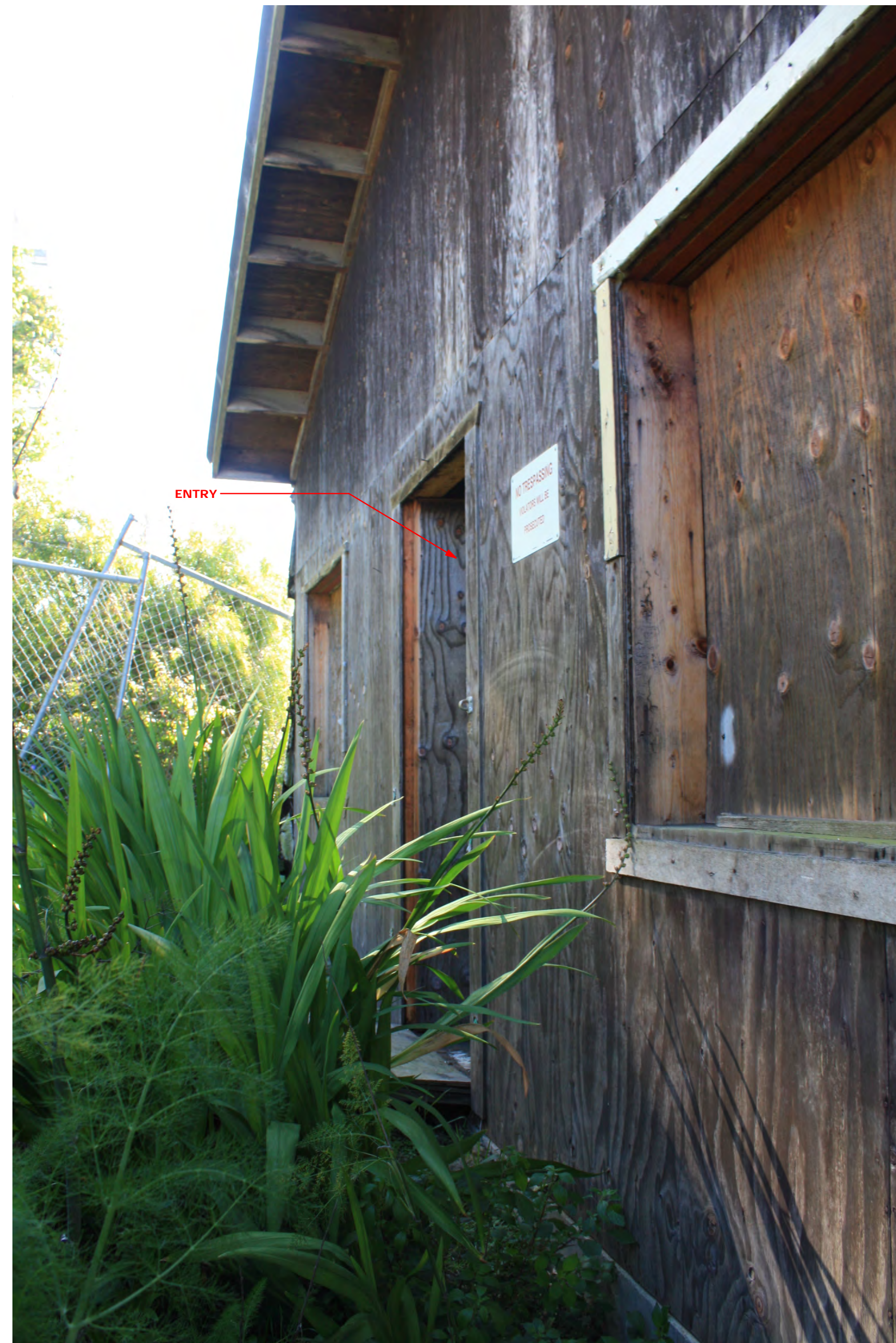
4 COTTAGE: EXISTING NORTH FACADE NOT TO SCALE
