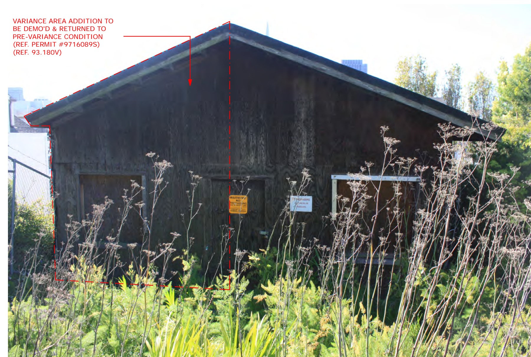
1 COTTAGE: EXISTING NORTH FACADE NOT TO SCALE
