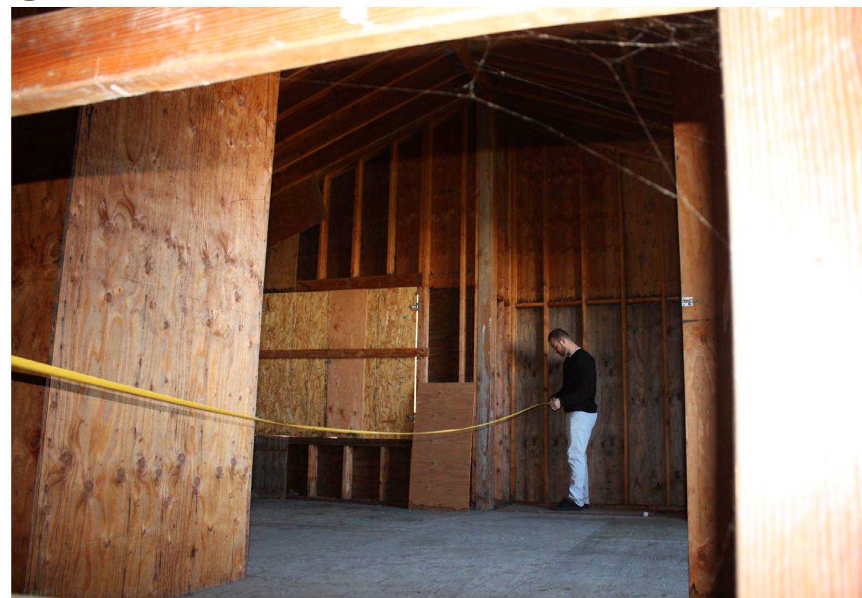
7 COTTAGE: EXISTING UPPER LEVEL LOOKING SOUTH NOT TO SCALE
