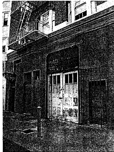
Figure 12 - 1649 Market Street, Stevenson St. detail
