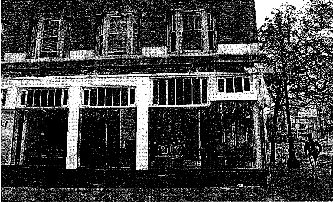
Figure 11 - 1649 Market Street, storefront detail
