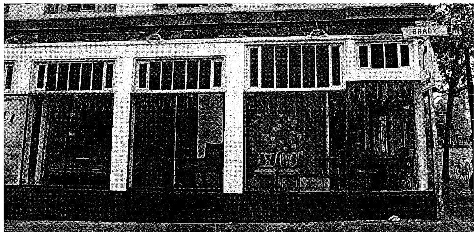
Figure 32 - 1649 Market Street, storefront detail
