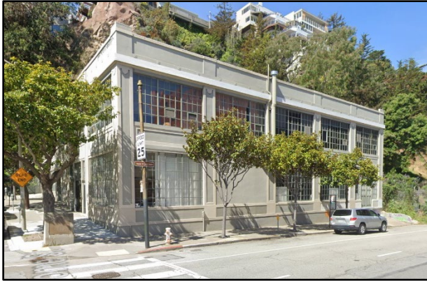
The Giusti Building/Farnsworth Lab at 202 Green Street was home to the first all-electronic "television system" and is California Landmark #941.
