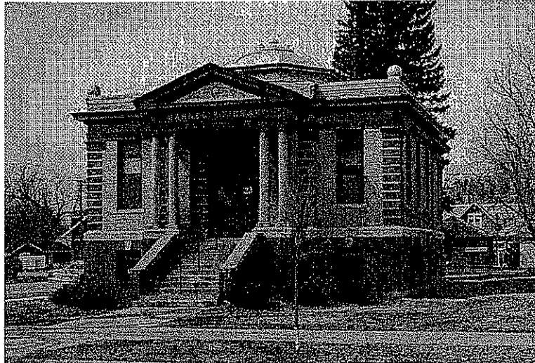
Figure 1. Typical Carnegie Library. Courtesy of the Library of Congress.
