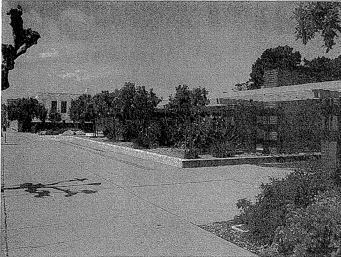
South Elevation of the Marina Branch Library.
