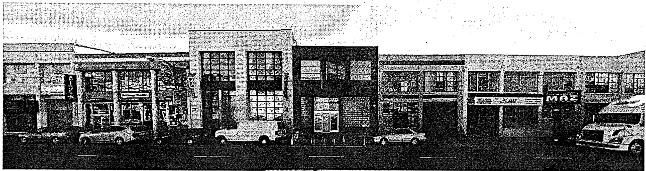
Bryant Street elevation. Photo by Google Maps
