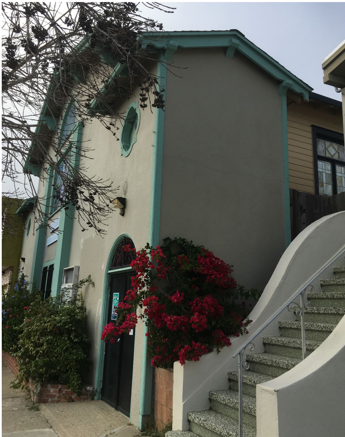
St. James Presbyterian Church, front (south) and east elevations, view northwest, 2022 Source: San Francisco Planning Department
