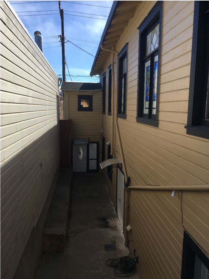
St. James Presbyterian Church, east elevation, 2022 Source: San Francisco Planning Department
