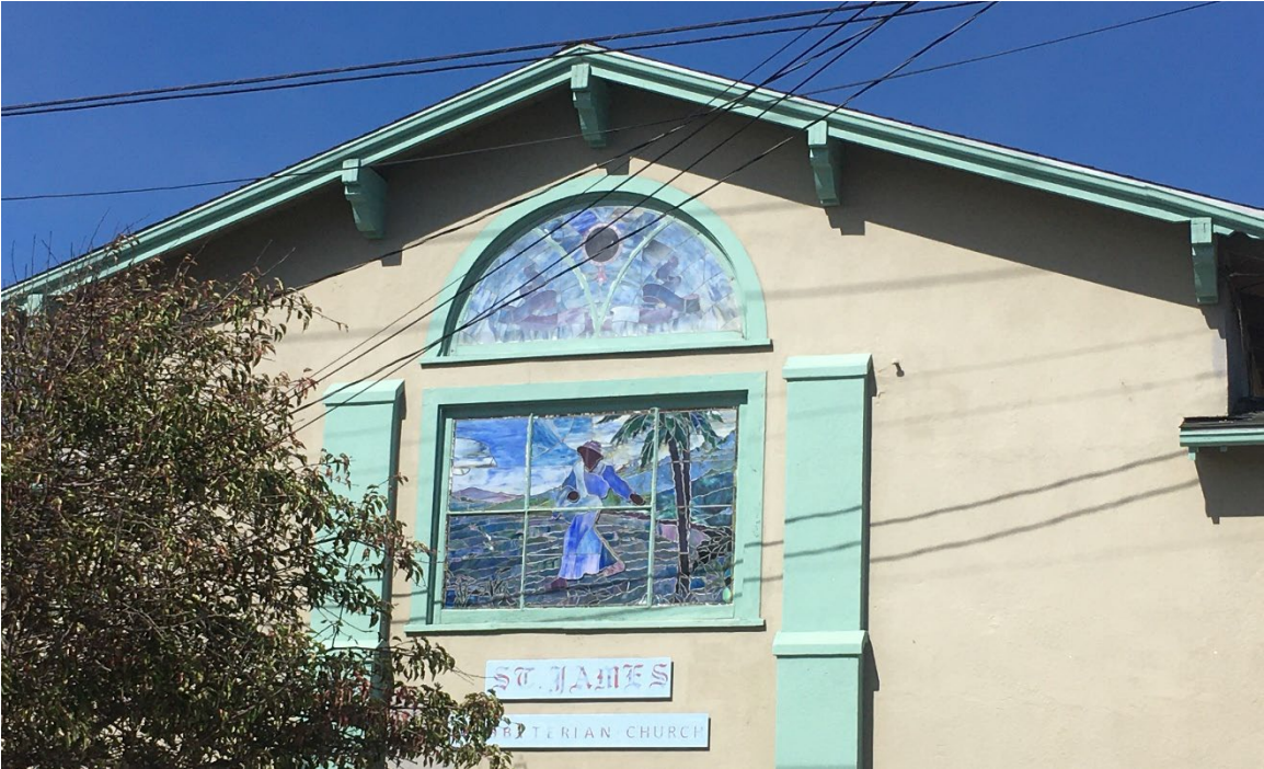
St. James Presbyterian Church, front (south) façade, stained glass, view north, 2022 Source: San Francisco Planning Department
