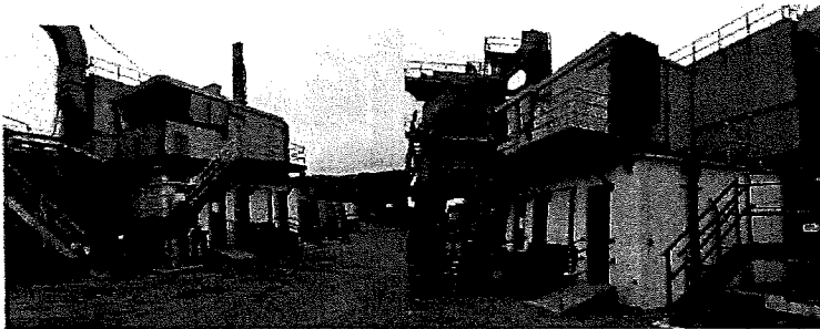
Electrical Power Room (bottom) and Control Room (top), northwest facing elevations (left) and southwest facing elevations (right)
