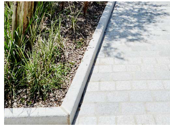
Curb at Sidewalk
