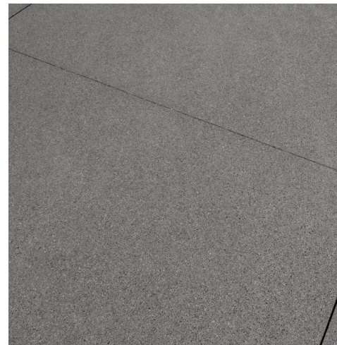
Paving waterjet concrete with integral color
