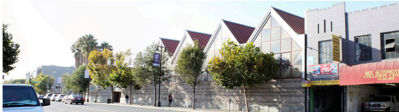
EXISTING CONDITION - 6TH ST
