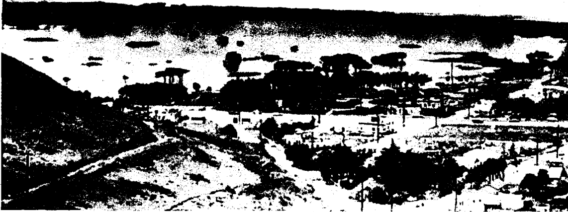
Figure 1 April 4, 1958 flooding of Sharp Park. Caused by storm water runoff and wave overtopping of berm. Geomatrix Consultants. Feasibility Study, Restoration of Coastal Embankment, Sharp Park Golf Course, Pacifica, California. November 1987. p. 20.
