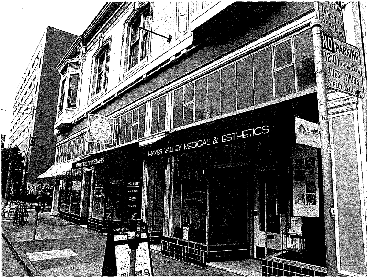
Figure 4 View of the commercial facades on Gough Street, viewed to the north-northeast.
