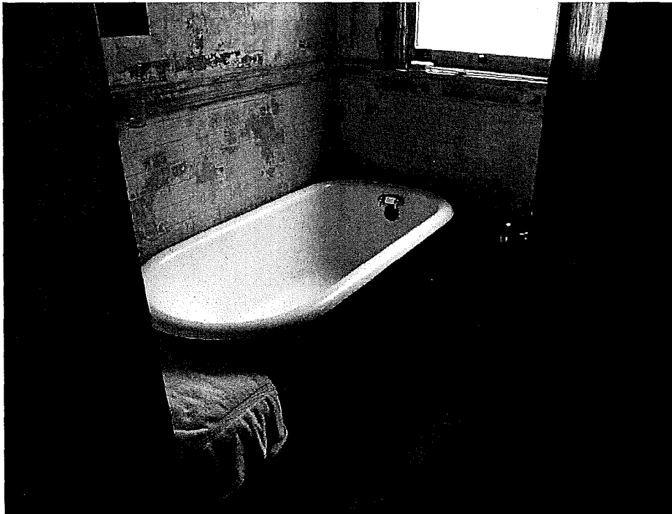
Figure 36 The bathroom in Rube Goldberg's apartment. The toilet is in a separate room from the bath room.
