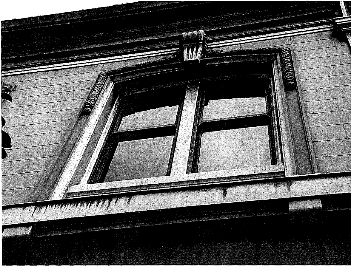
Figure 11 Primary façade window with Beaux Arts decorations of garlands, shaped keystone, and curved lintel. Two sets of paired windows in this form center the second stories of both the Gough Street façade and the Oak Street elevation.
