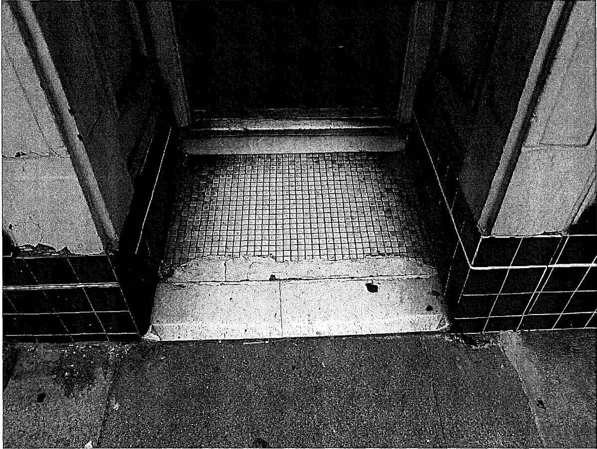
Figure 6 The marble threshold tread with white square mosaic vestibule floor at 194 Gough Street.
