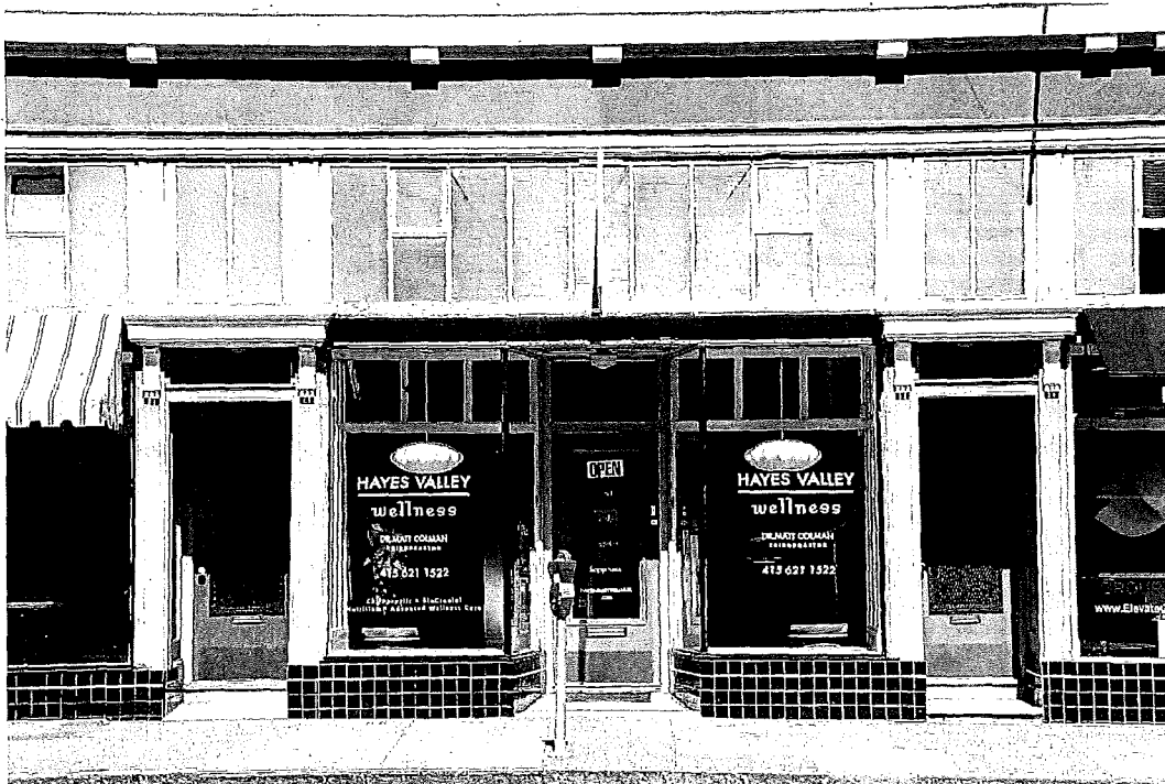
Figure 8 The commercial facade of 188 Gough Street flanked by the residential entrances to 194 Gough St. (left, Rube Goldberg's residence) and 186 Gough St. (right, Max Goldberg's residence).
