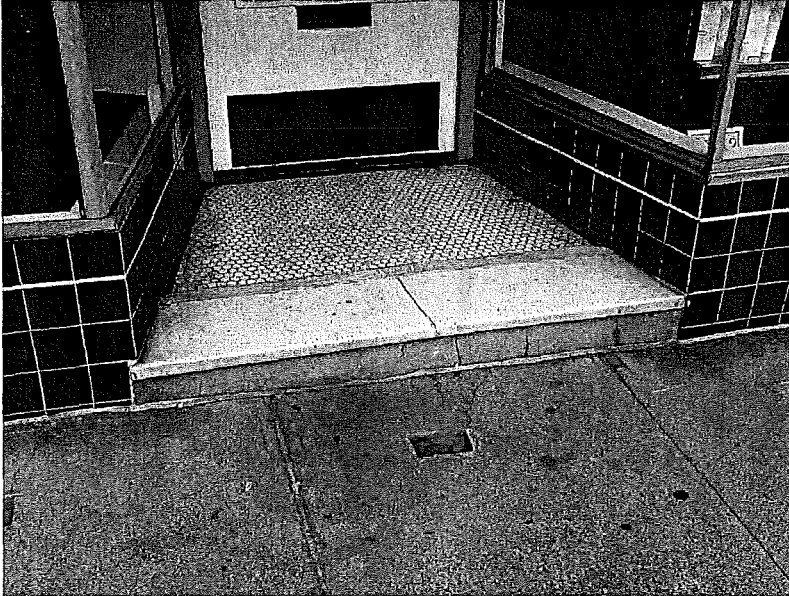
Figure 17 Original marble step and mosaic tile landing at 190 Gough Street. All five thresholds on the façade retain their original marble and tile finishes. Note the black tile with weather course that runs the length of the façade.
