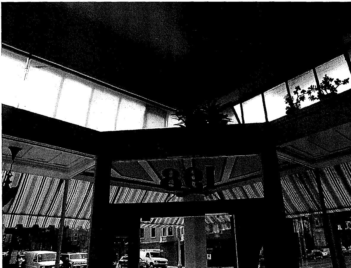
Figure 39 Interior view of the corner commercial space at 198 Gough Street at the corner of Oak Street. Note original finished carpentry on the ceilings of the display area and transom windows of the former saloon. Some doorway framing has been replaced in-kind in a recent rehabilitation by the current tenant.
