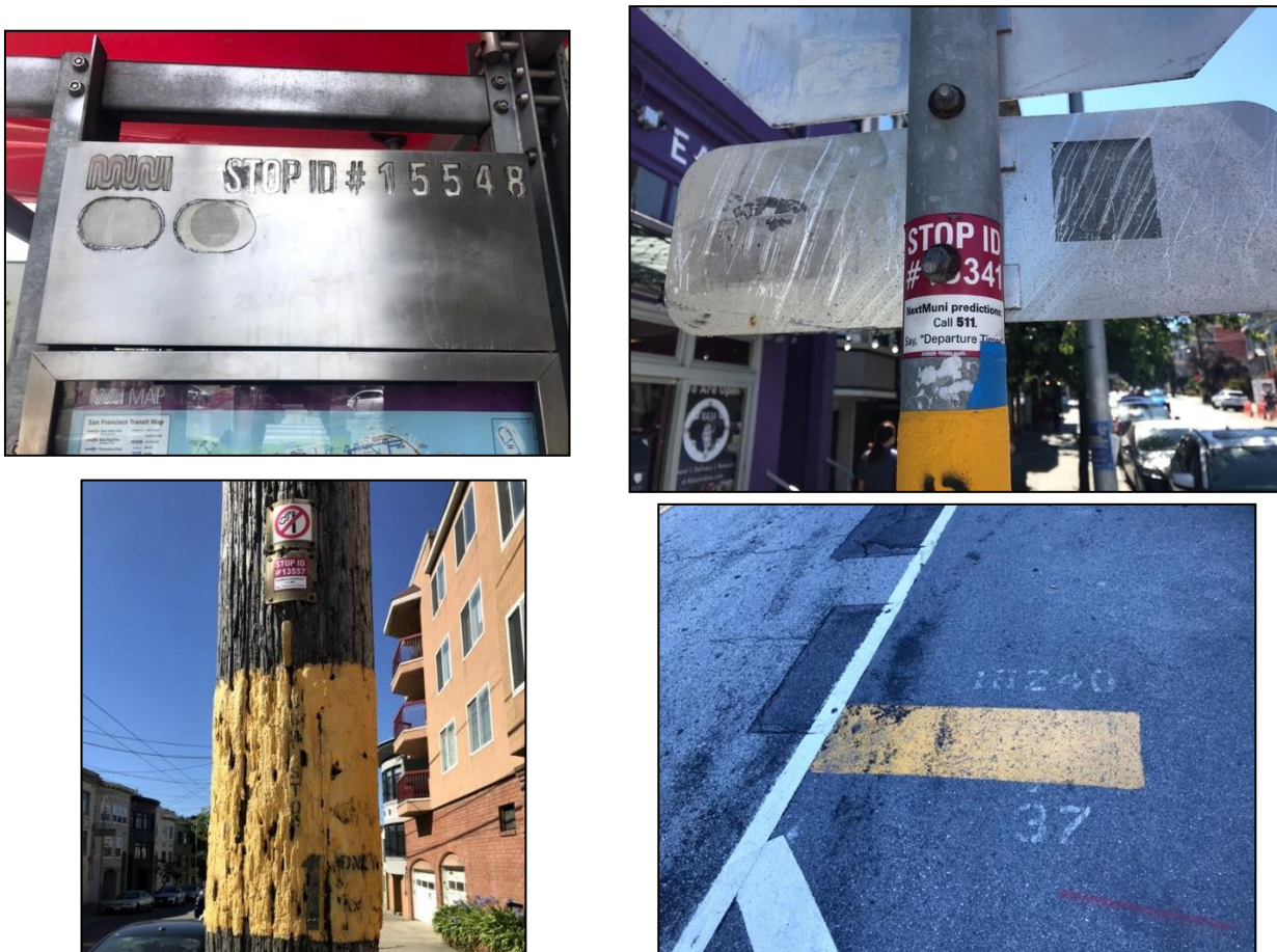
FIGURE 6. Examples (clockwise from top left) of shelter markings worn out from the sun, obscured NextBus ID stickers, telephone poles with difficult-to-read lettering, and worn out pavement paint
