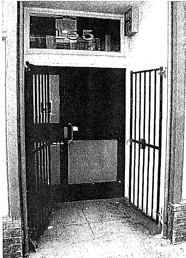
Figure 1. Metal entry door at west elevation.
