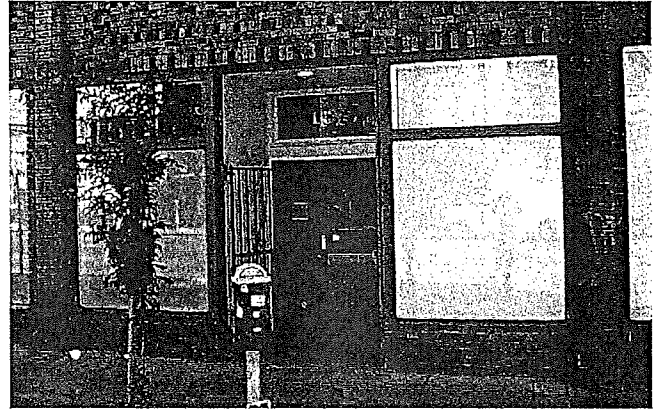
Figure 1. Storefront at west elevation.
