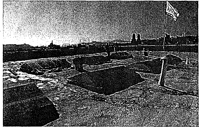
Figure 1. Roof overview; note skylights.
