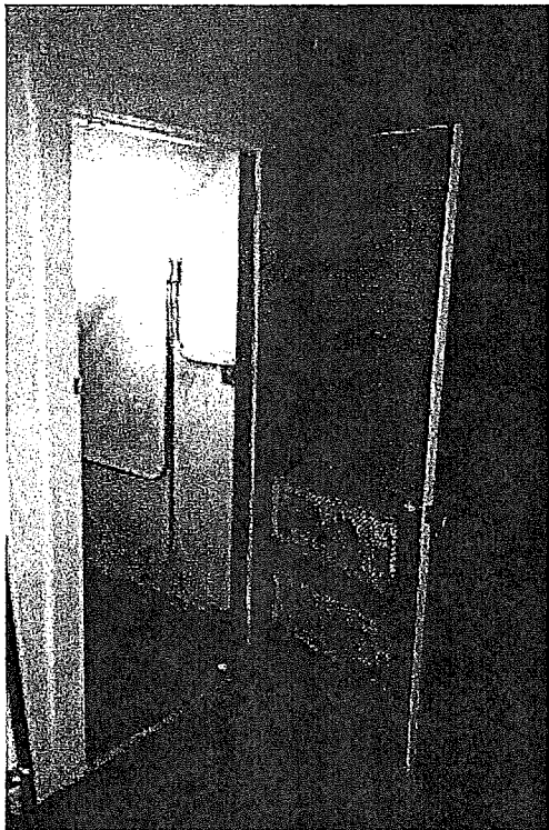
Basement entrance with original door. (Page & Turnbull, April 2013)
