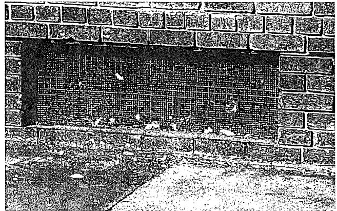
Figure 1. Ventilation grilles; note 1"x1" historic iron grille.
