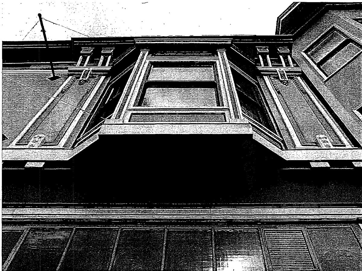
Figure 13 The living room designed for Max Goldberg was illuminated by this bay window on the southern end of the west facade at 186 Gough Street. The paneled pilasters on either side of the fenestration topped with garlands and paired brackets create the illusion of a projecting wing and emphasize the symmetry of the façade because the feature is repeated at the north end of the façade. Note the relieved cornice molding that contributes to the illusion of the end feature's projection.
