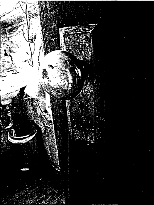
Figure 34 Hardware of brass and bronze from 1911 remain in the residential and much of the commercial units of the building.
