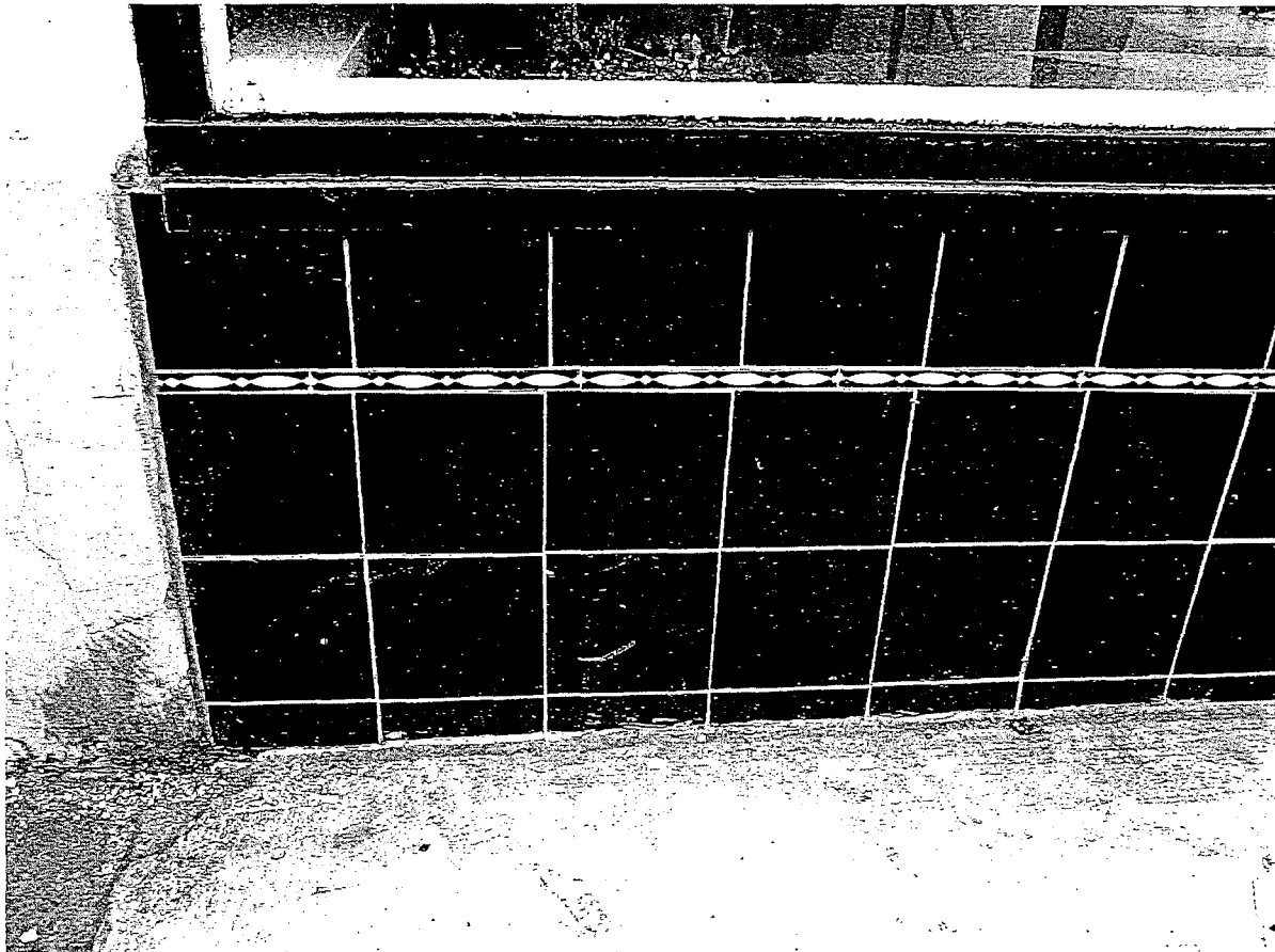
Figure 5 Black tile bulkhead with lozenge and bead narrow course as seen here at the east end of 198 Gough Street's commercial facade on Oak Street.
