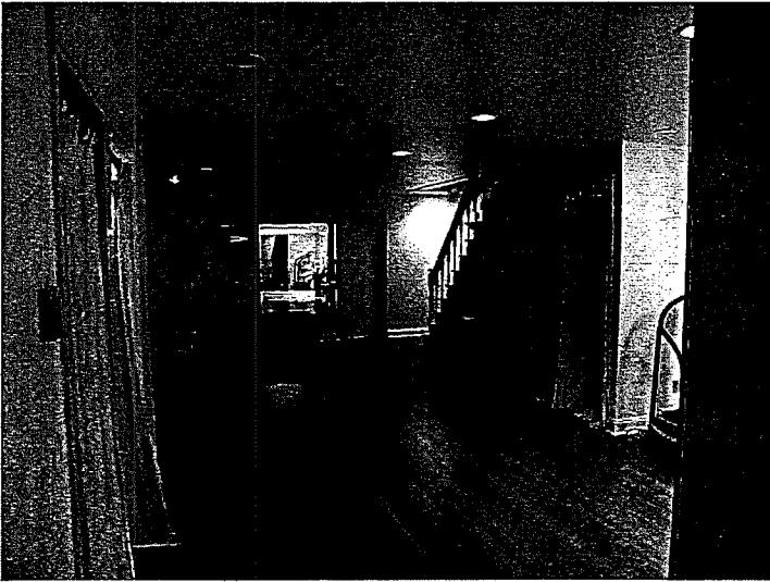
Figure 44 The basement of the central commercial unit, 190 Gough Street, has been finished in drywall. Original stair balustrade and wood door surrounds were left in place.
