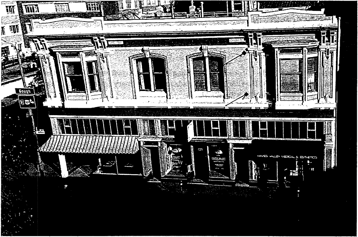
Figure 2 .The Gough Street, west façade of the R. L. Goldberg Building.
