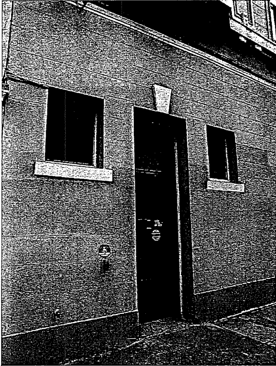
Figure 20 Service door at the east end of the Oak Street elevation. The door is topped by a keystone and flanked by high-set square windows with prominent sills.
