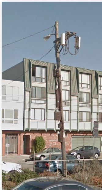
Crown Castle, for Verizon Wireless “oDAS XL” Personal Wireless Services Facilities, in the Outer Sunset. The bulky nature and potential noise generation from cooling fans on residential streets is disfavored.
