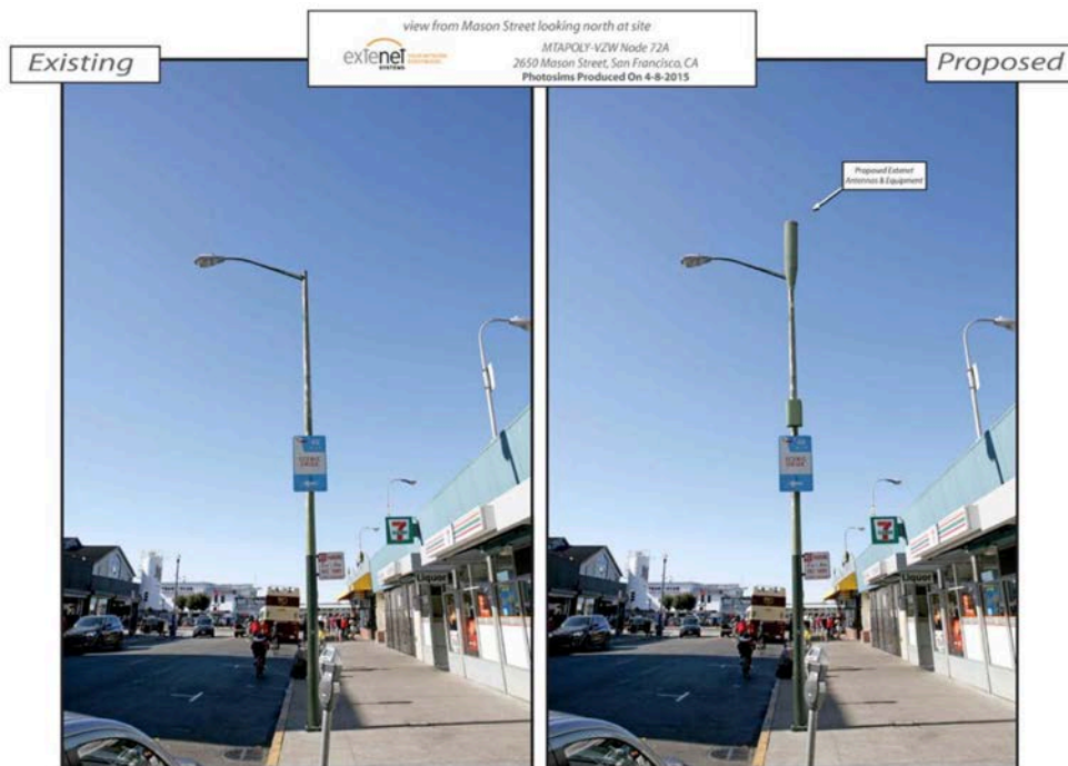
Extene! Systems, for Verizon Wireless “oDAS R” (or Small Cell) on a steel light pole owned by the City (SF Public Utilities Commission). An antenna is located on top and two computers (equipment) are located midway down the pole. Planning Department staff worked with the Department of Public Works, and the carrier to create a bracket to “screen” one of the computers with road signage.
