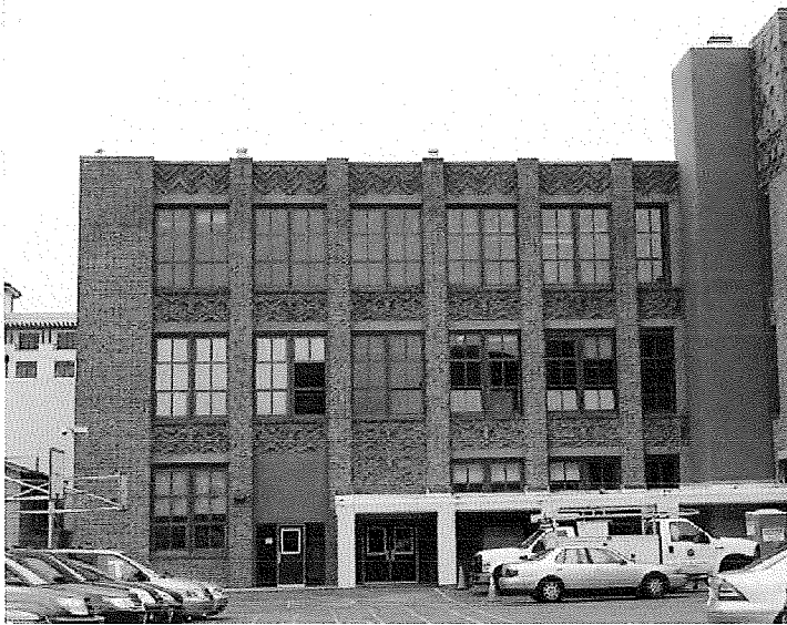
Figure 33. North façade of gymnasium wing of Theodore Roosevelt Middle School; view toward south.
