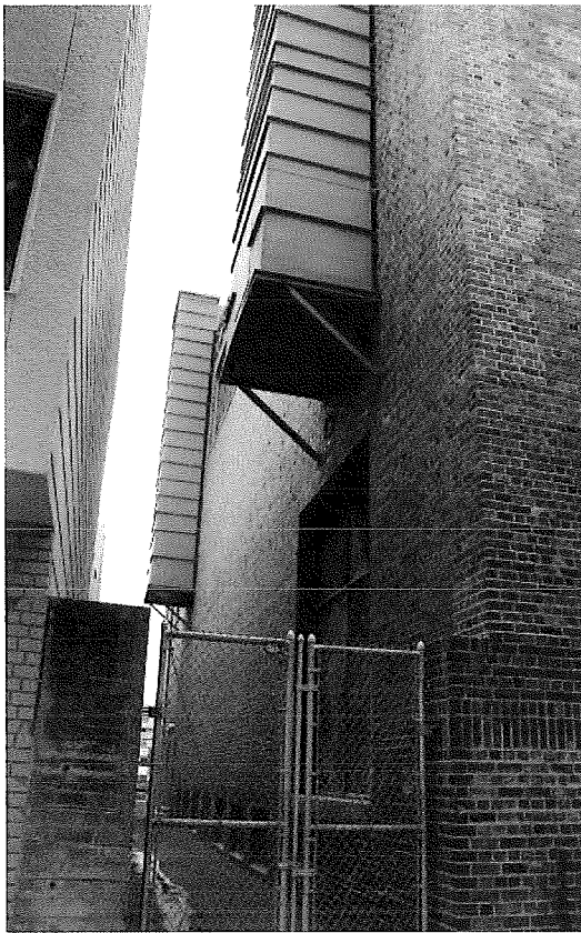
Figure 34. North façade along north property line; view toward east.
