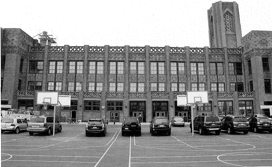
Figure 29. Central section of east façade of Theodore Roosevelt Middle School; view toward west.
