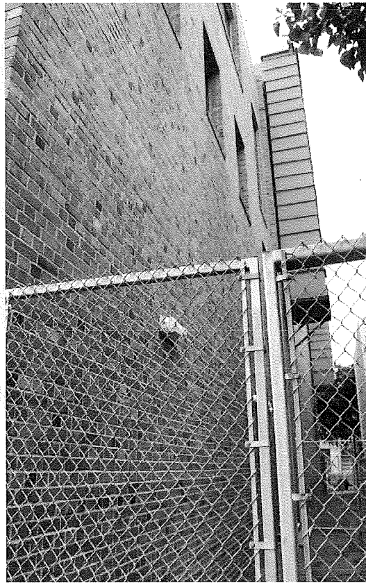
Figure 35. North façade along north property line; view toward west.
