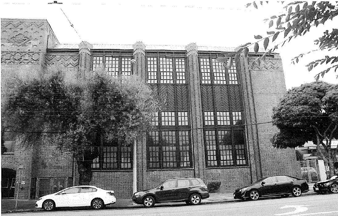
Figure 26. West façade of gymnasium wing.
