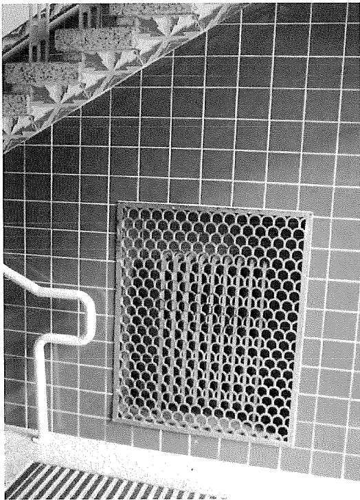
Figure 44. Tiled wainscoting and decorative metal radiator screen.
