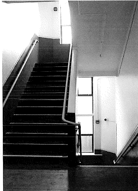
Figure 45. South stair between second and third floor levels.
