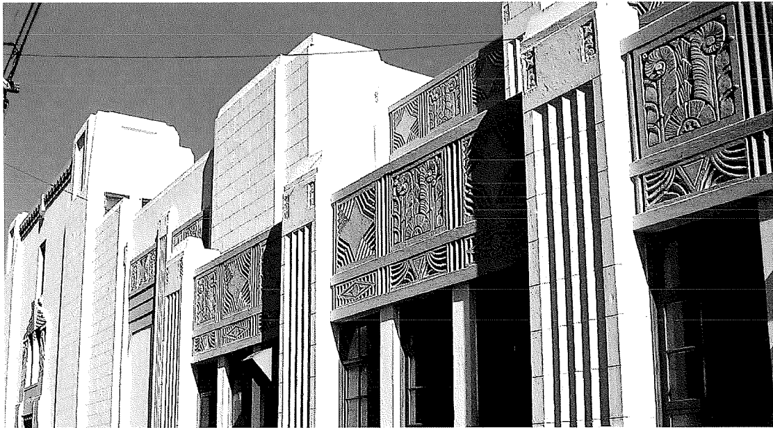
Figure 80. Detail of James Lick Middle School, by William H. Crim, Architect.
