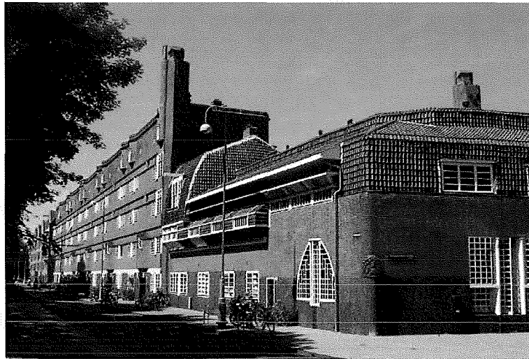
Figure 82. "Het Schip," Amsterdam, by Michel de Klerk, Architect.
