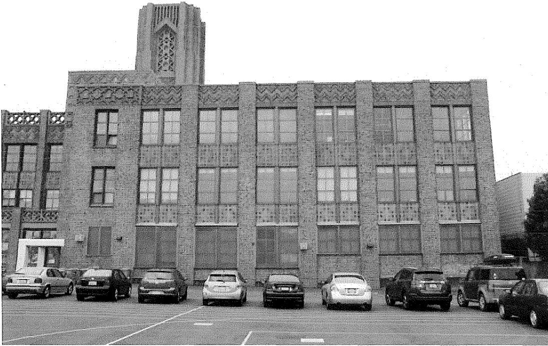
Figure 30. North section of east façade of Theodore Roosevelt Middle School; view toward west.
