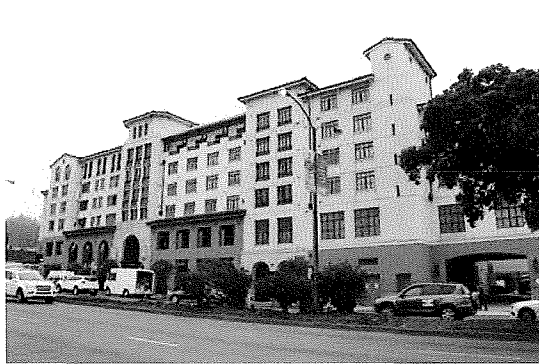
Figure 8. 3575 Geary Boulevard, constructed 2011; view toward southeast.
