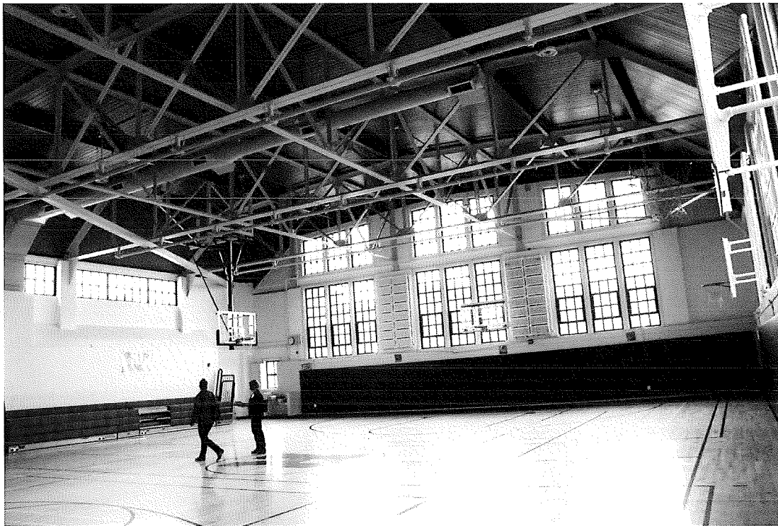
Figure 53. Upper gymnasium, third floor.
