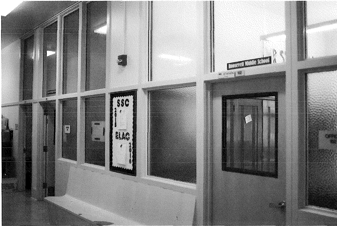
Figure 47. Windows and bench in administration office suite.
