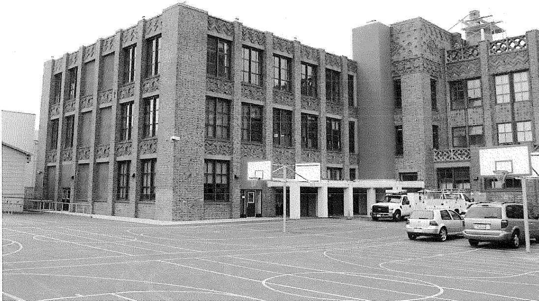
Figure 28. East façade (south section) of Theodore Roosevelt Middle School; view toward southwest.
