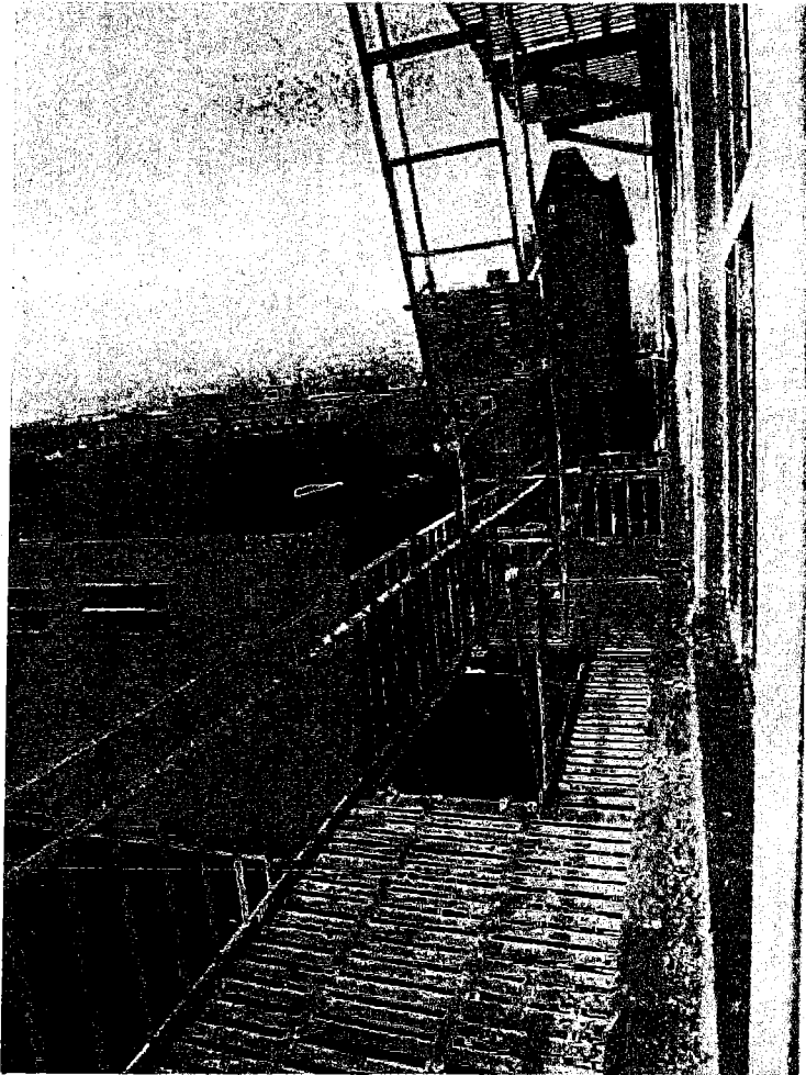
Fire Escape at Stevenson Street Facade
