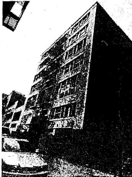
Stevenson Street Facade (Southeast Corner)
