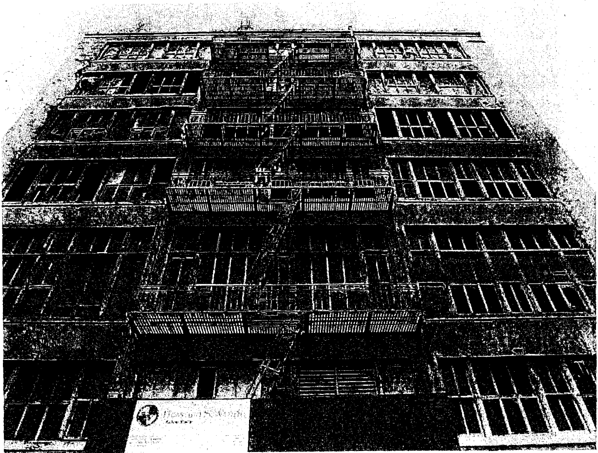
View of Stevenson Street façade looking up
