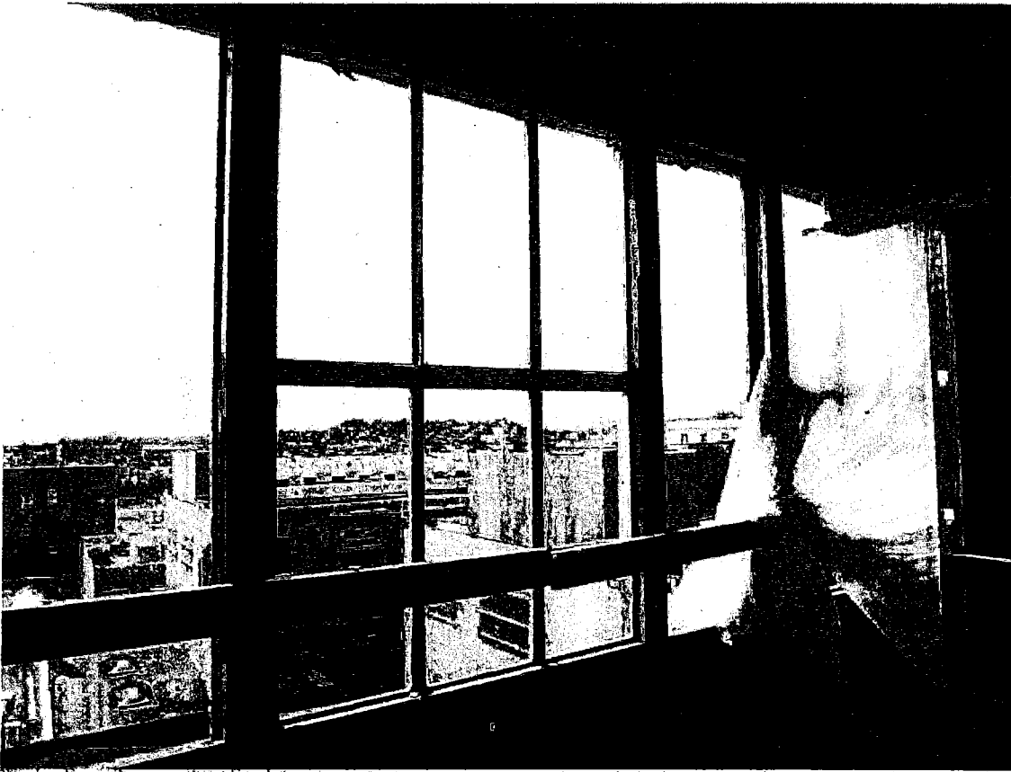
Window Frame Stevenson Street Facade from interior
