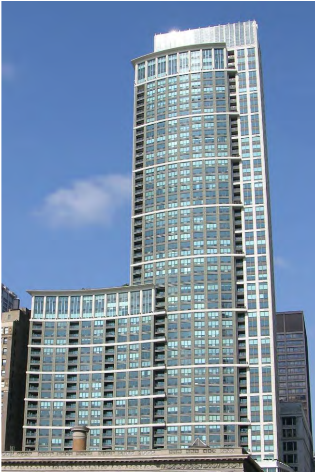
Heritage at Millennium Park
