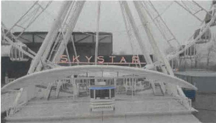
Figure 12: The base of the SkyStar Observation Wheel, including ticket booth and canopy. Accessibility ramp partially visible on the left of image.
