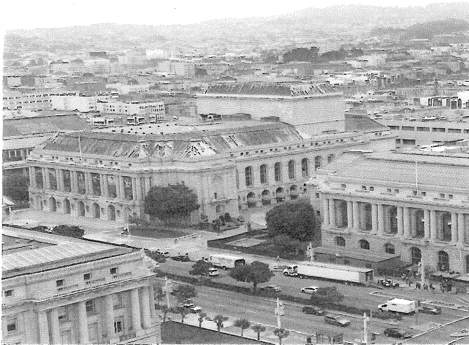
Opera House Roof: Solar PV System to be installed on flat roof; Mansard/sloped roof to be replaced.
