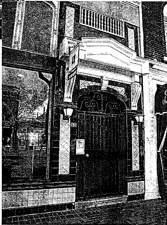
Figure 22 - 1670 Market Street entry detail
