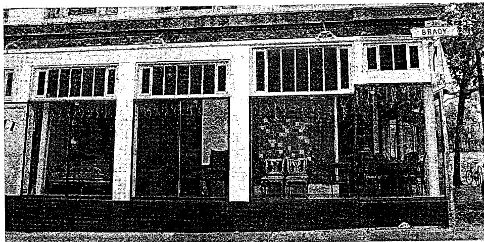
Figure 32 - 1649 Market Street, storefront detail
