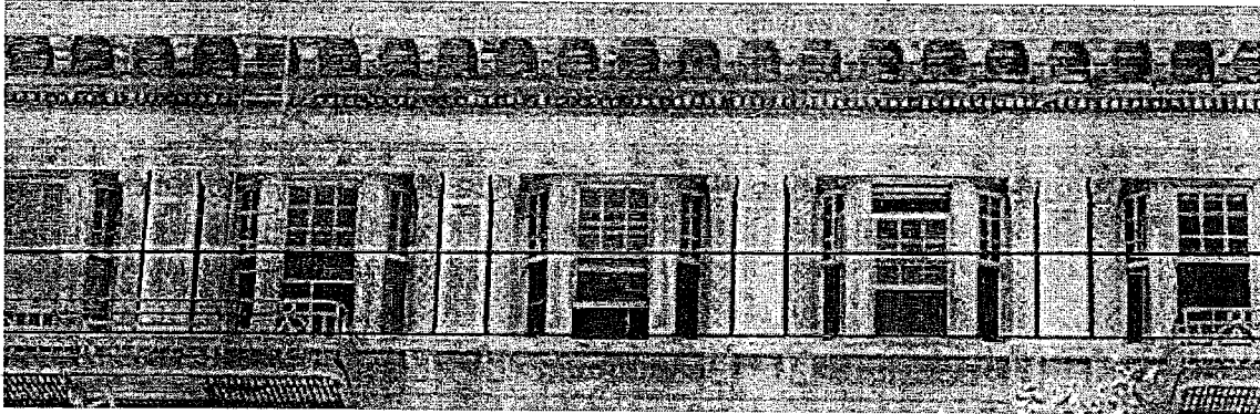
Figure 31 - 1649 Market Street, terra cotta 5th floor and metal entablature detail
