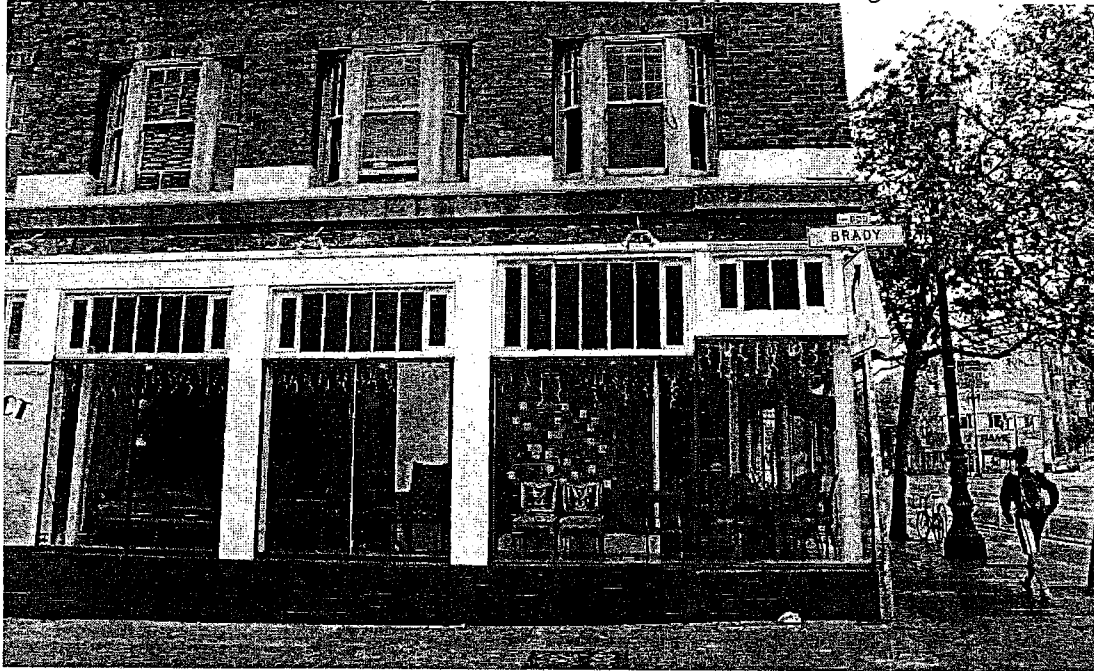
Figure 11 - 1649 Market Street, storefront detail
