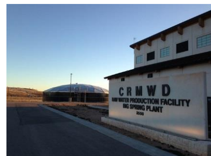
A team led by Carollo was selected by the Texas Water Development Board to perform a comprehensive evaluation and monitoring study of the Raw Water Production Facility in Big Spring, TX, the country's first direct potable reuse facility
