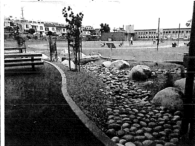
Downspout flowing into infiltration trench (RL Stevenson Elementary, San Francisco)
