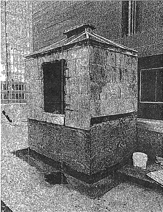
Figure 48: Photograph of elevator penthouse clad in metal panels over wood sheathing. Note surface corrosion on metal panels and missing access door (photograph taken on 02/27/2018)
