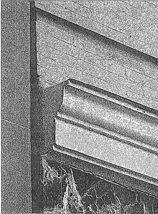
Figure 16: Detail photograph of sheet metal water table banding at second floor. Note brick erosion beneath the paint on the brick substrate (photograph taken on 01/26/2018).
