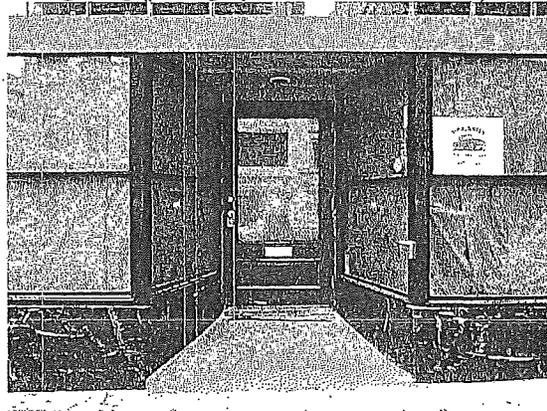
Figure 13: Photograph of the third bay entry from south end with angled storefront glazing system, paneled wood door, wood panel ceiling, and marble cladding (photograph taken on 01/26/2018).
