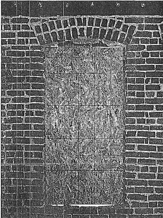
Figure 33: Detail view of typical punched window opening at western wall. Note arched brick lintel (photograph taken on 02/27/2018).
