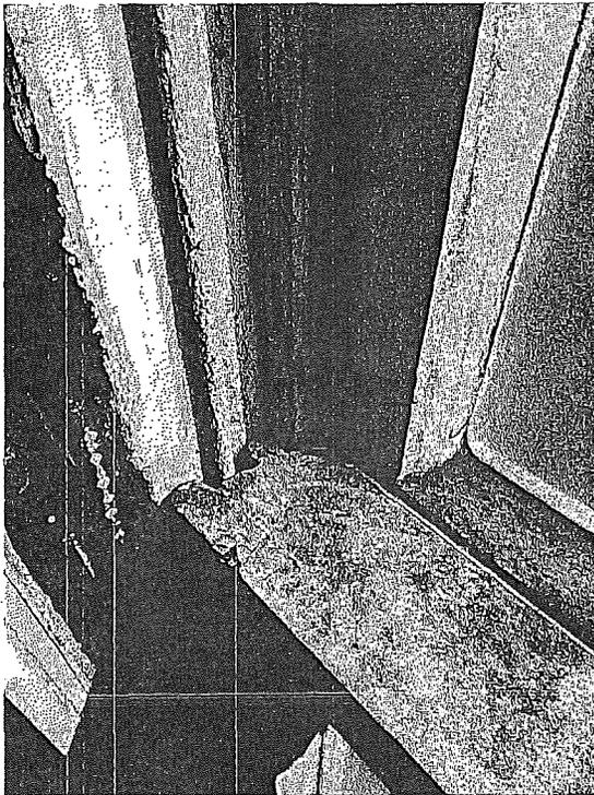
Figure 43: Detail photograph of top edge of lower sash, and sash cord. Note typical paint chipping and missing sash stop (photograph taken on 02/27/2018).
