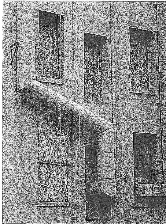
Figure 22: Detail photograph of ventilation ducts projecting through second floor openings. Note size difference between window and door openings (photograph taken on 01/26/2018).
