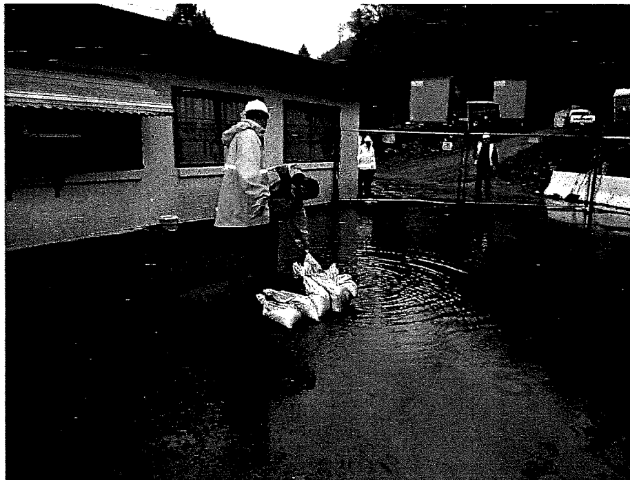
Figure 5. Flooding inside Switchyard near control building (2/28/2014).
