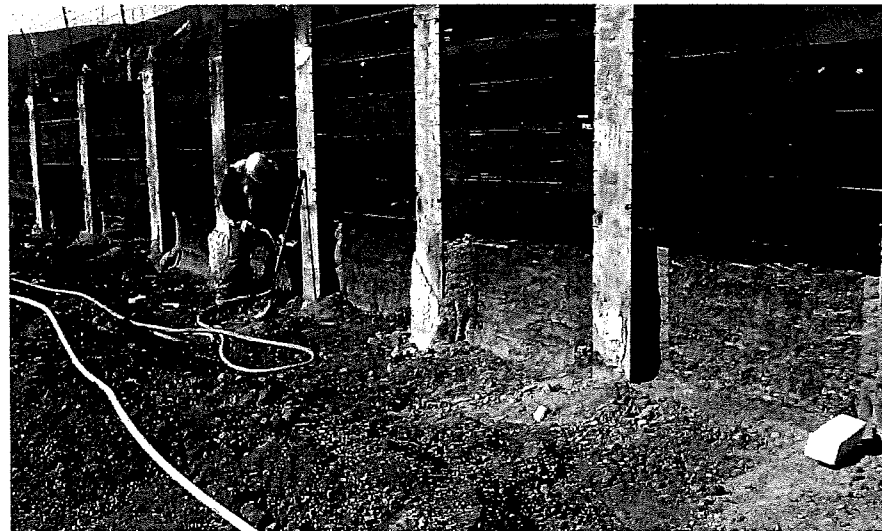
Soldier Pile and Lagging Retaining Wall Construction
