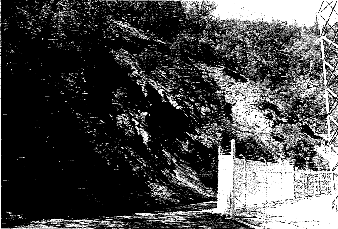
Figure 2-4: Work Area 1 – Active Slope Failure at East End of ISY (May 2, 2014)
