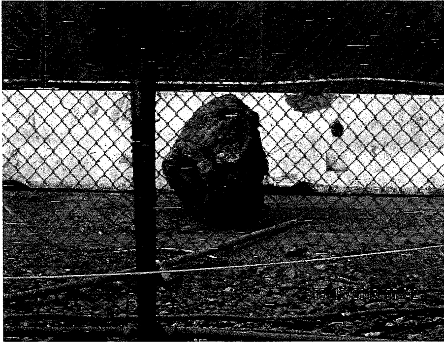
Figure 2. Boulder that traveled over/through temporary safety fencing and came to rest on the access road behind the Switchyard (9/10/2013).
