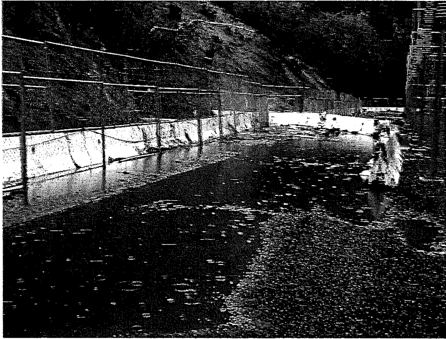
Figure 4. Flooding inside the Switchyard after rain event (2/28/2014).
