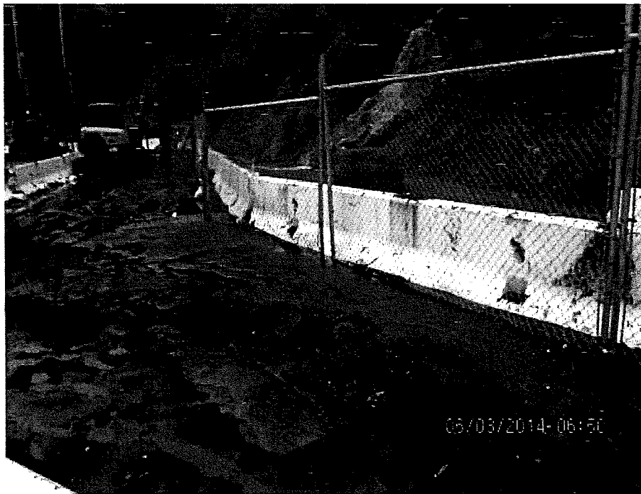
Figure 7. Mud and sediment build up after rain event (3/6/2014).
