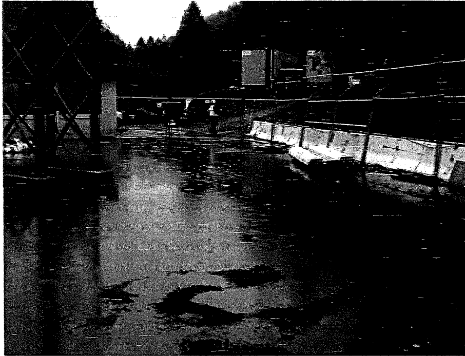
Figure 6. Flooding inside Switchyard near control building (2/28/2014).
