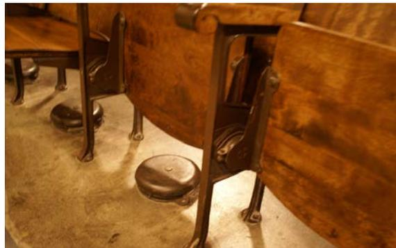
Figure 41. Heating units beneath seats.
