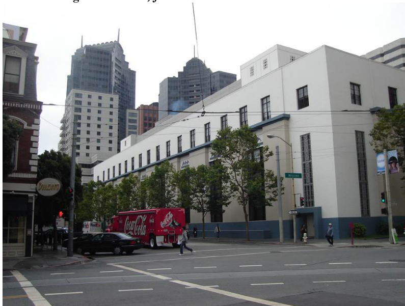
Figure 19. West side of Stuart Street, looking southwest from Mission Street.
