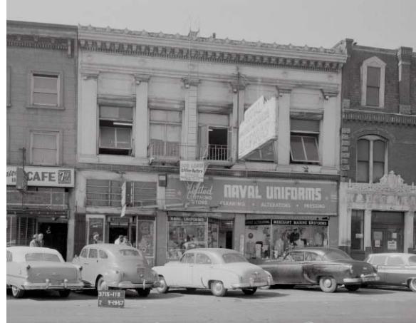
Figure 8. 110 The Embarcadero, 1957. Source: San Francisco History Center, Assessor's Office Negative Collection, sfp- 23_block_box2_block#3715_no.g10_on_strip
