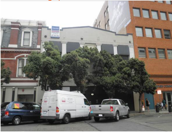
Figure 10. 113-115 Steuart Street. Source: Page & Turnbull, August 2013.
