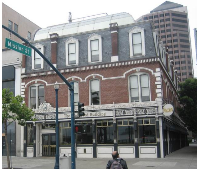
Figure 21. Audiffred Building (1889). View west from The Embarcadero. Source: Page & Turnbull, June 2007.
