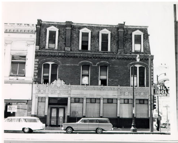
Figure 9. 110 The Embarcadero (partial view on left), 1964. Source: San Francisco Historical Photograph Collection, AAC-5090.
