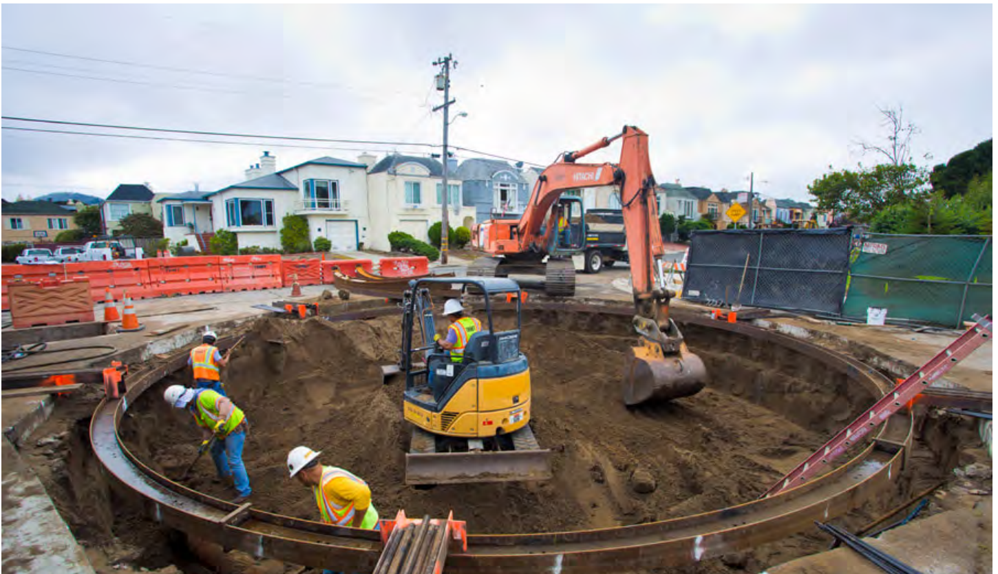
Emergency Firefighting Water System cistern construction
