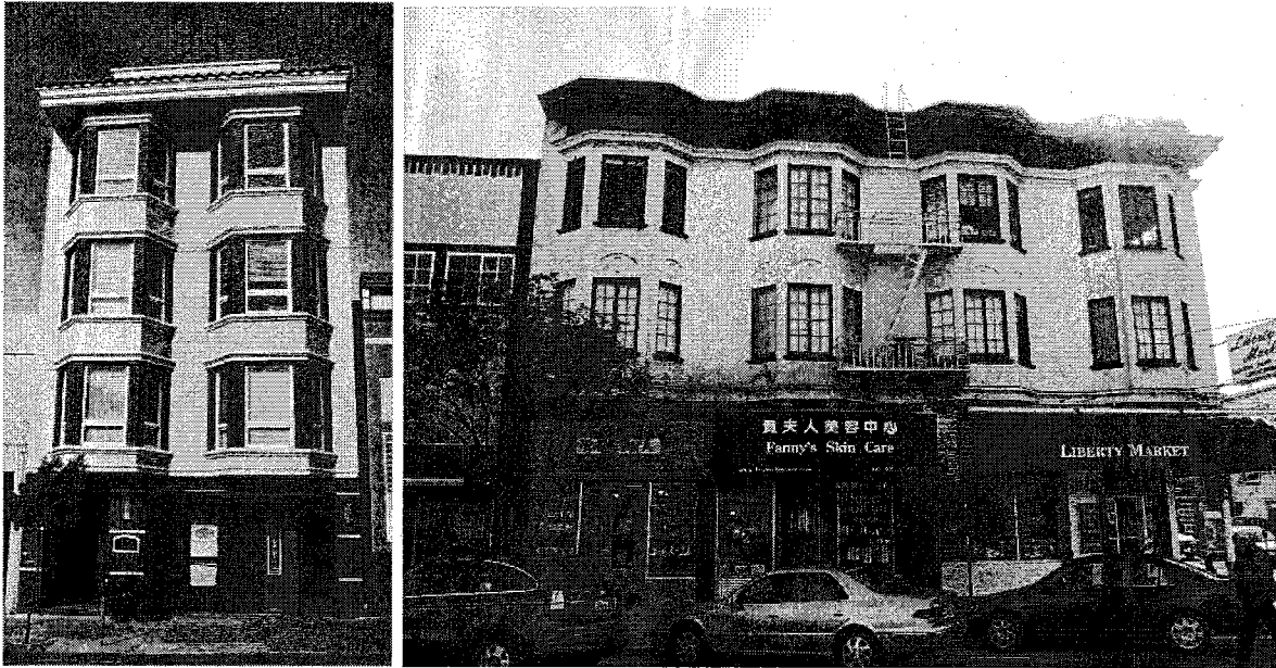
Figure 2-The building on the left is located on Geary Boulevard and 2 nd Avenue and demonstrates a new development under 40-X including three floors on top of a low ceiling, inactive ground floor. In contrast, the building on the right, located on Geary Boulevard and 23 rd Avenue is almost the same height and is able to provide a generously high ceiling and active ground floor.
