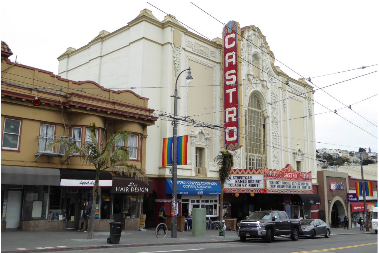
Front façade, from northwest. Image Source: Page and Turnbull, 2019
