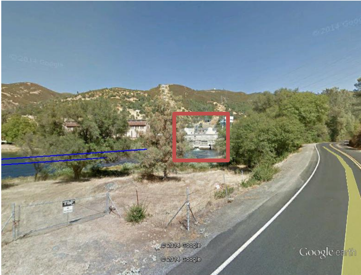
View from State Highway 49 facing Southeast Powerhouse in Center of Image Google Earth Image Dated July 17, 2014
