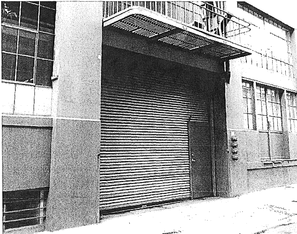
A6. View of the loading dock along the north façade, looking south (ARG, October 2015).
