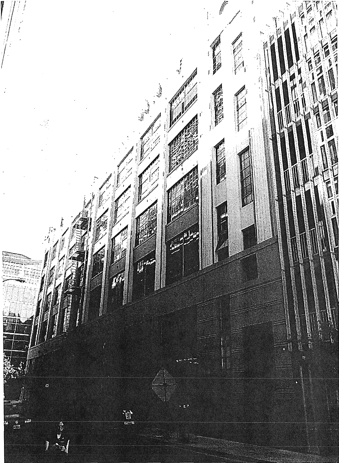
A3. View of north façade, looking east (ARG, October 2015).
