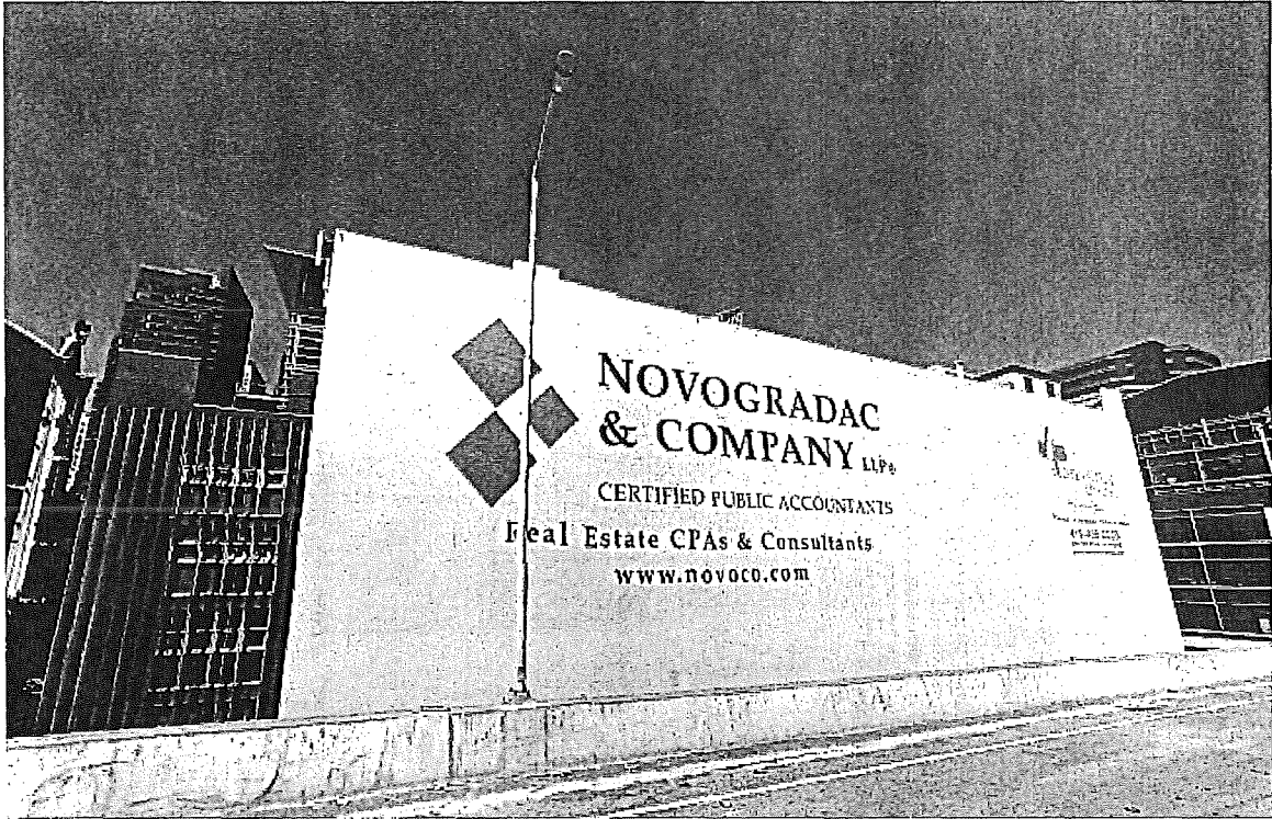
A9. View of south façade, looking north (Google street view, accessed October 2015).
