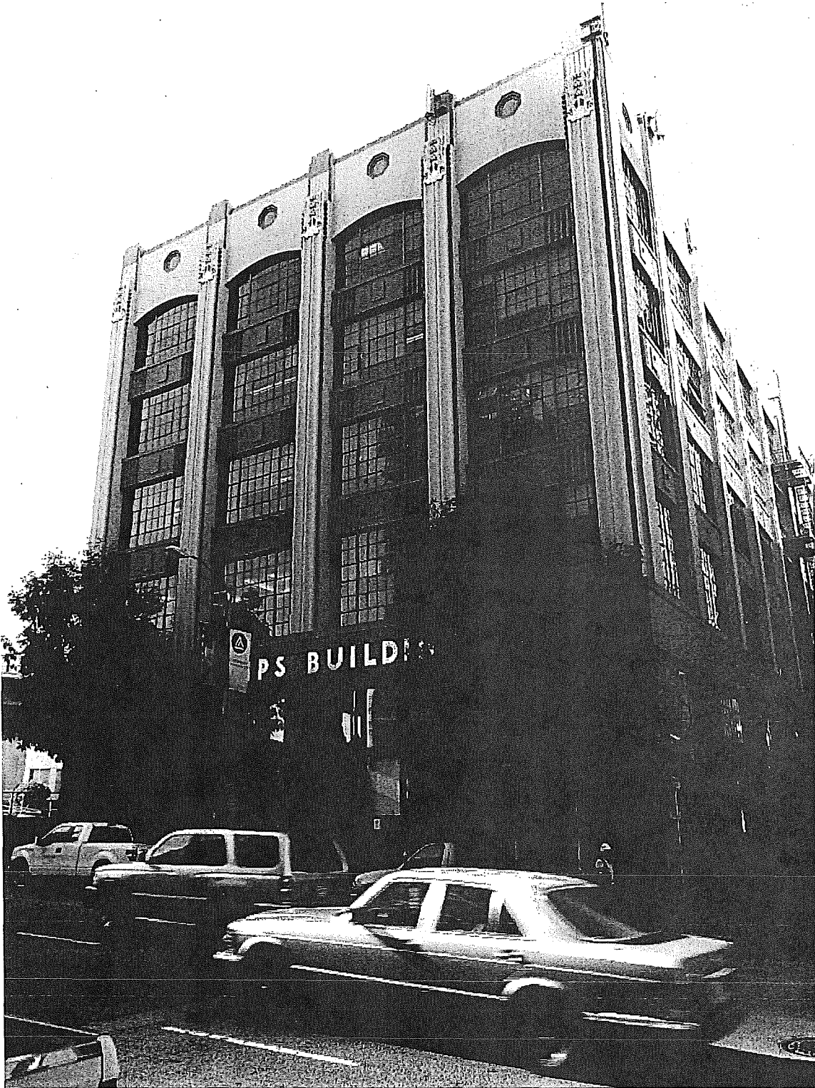
A1. View of front (east) façade, looking south (Architectural Resources Group, October 2015).
