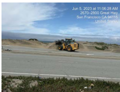
Loader south of Taraval piling sand from road onto the area next to the road shoulder. 10:50 AM 6/5/23.
