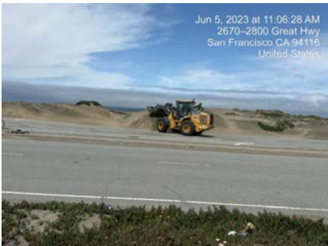
Loader south of Taraval piling sand from road onto the area next to the road shoulder. 10:50 AM 6/5/23.
