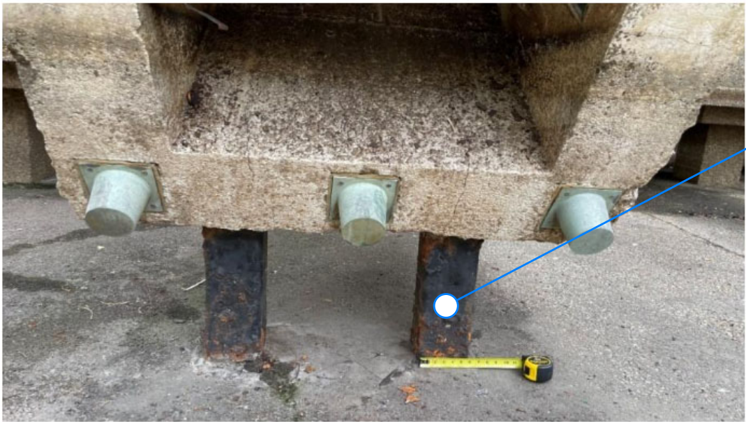
Figure 8: Vaillancourt Fountain - Corroded Steel Tubes and Spalled and Cracked Concrete
