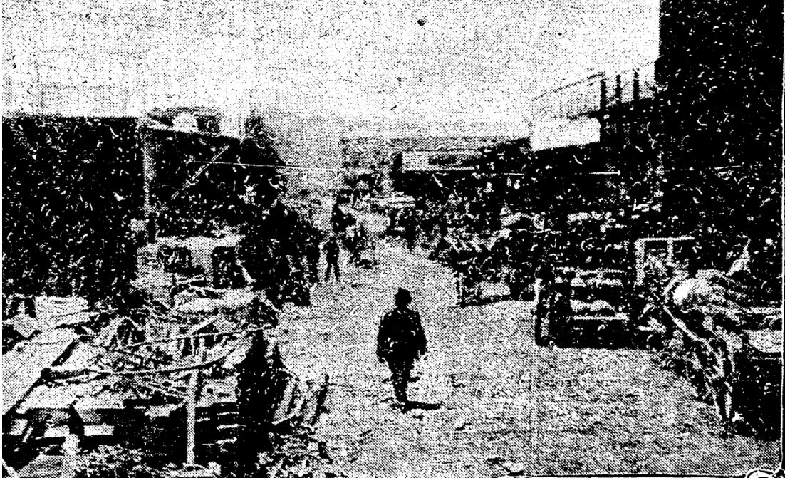
Rebuilding the Commission District. Source: San Francisco Chronicle , June 28, 1906
