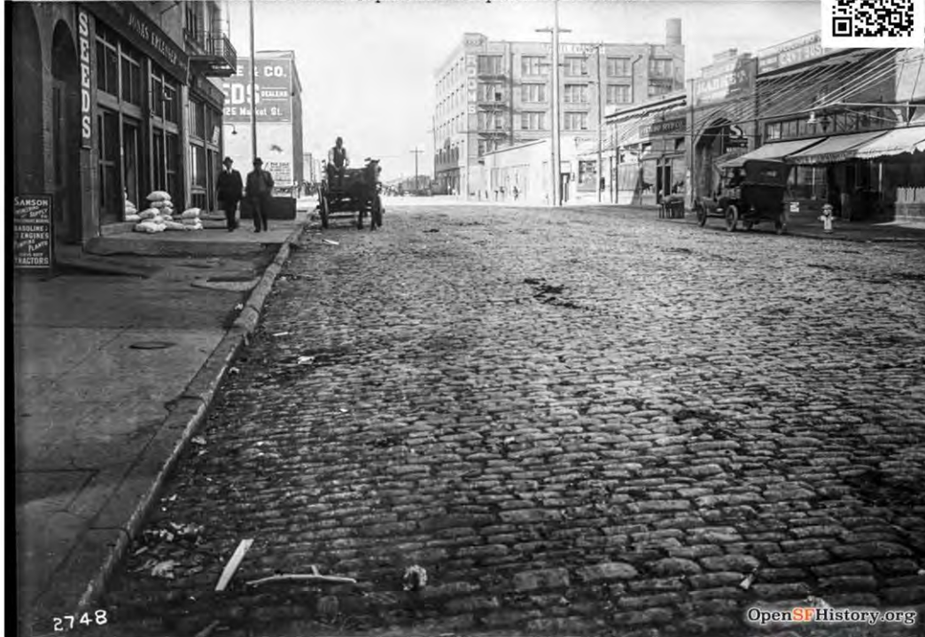
Front Street apparently suffered greater damage, as a photo taken in 1915 shows only the arch (extant) with newer storefront windows with transoms instead of arches. Source: OpenSFHistory / wnp36.01003.
