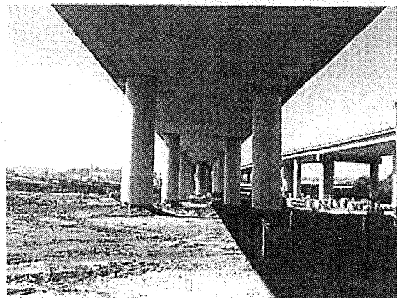
Parcel No. 1 freeway bents
