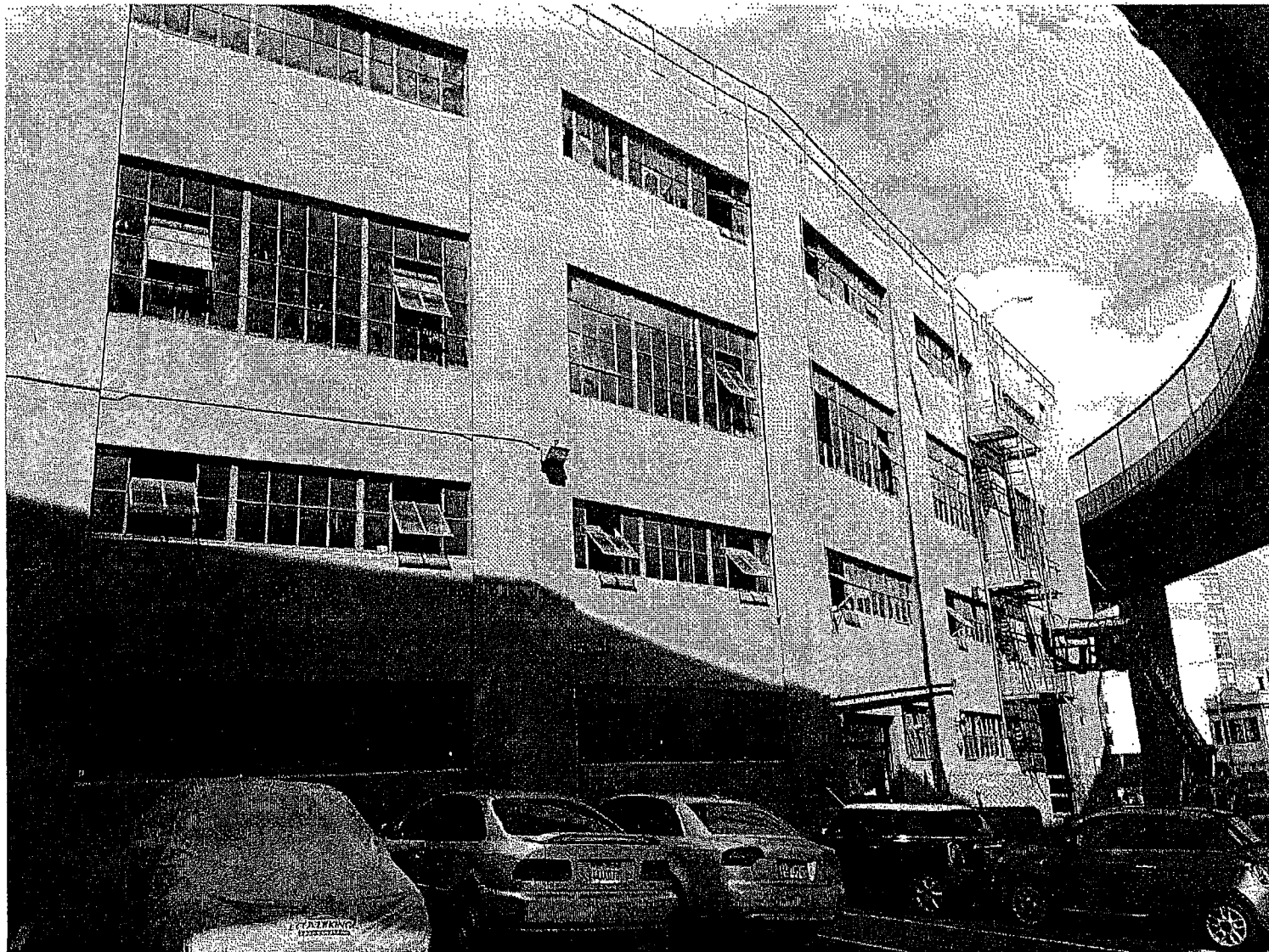
Photo 5: Project site viewed from the adjacent Caltrans-owned parking lot, looking east. Westbound I-80 Harrison Street off-ramp viaduct is visible in the upper right. – March 28, 2014
