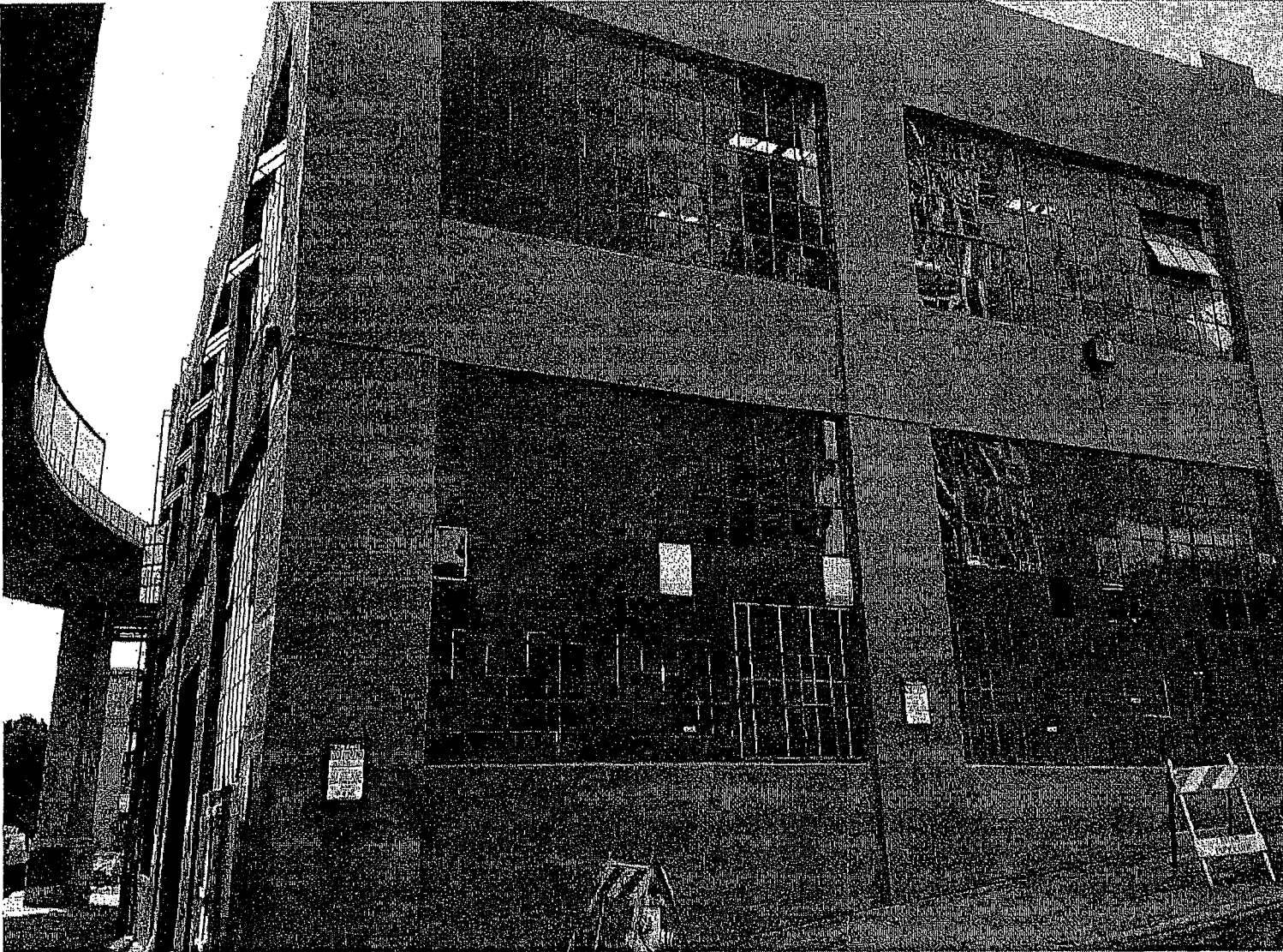
Photo 4: Project site viewed from Rincon Street, just north of Bryant Street, looking west. Westbound I-80 Harrison Street off-ramp viaduct is visible in the upper left. – March 28, 2014
